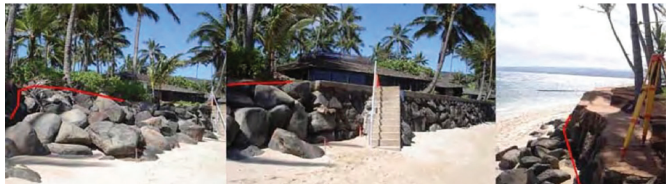
Photos taken in July 2007 of the Dailey seawall and portions of the revetment that were not improved. CREDIT: ENVIRONMENTAL ASSESSMENT FOR SHORELINE SETBACK VARIANCE.
