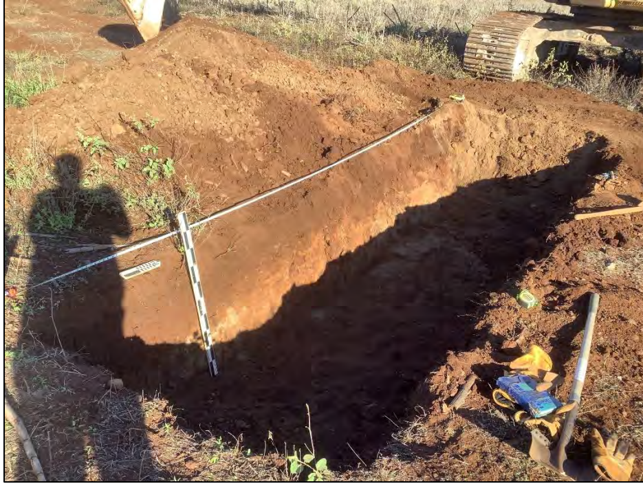
Figure 22. TE-1, general view of west wall, view to northwest
