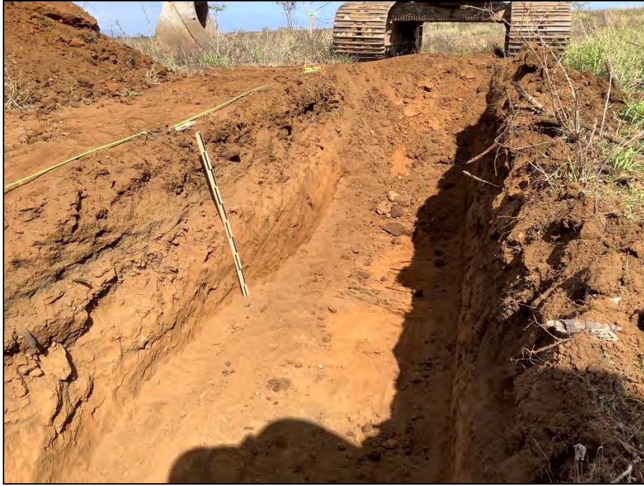
Figure 52. TE-11, general view of west wall, view to north
