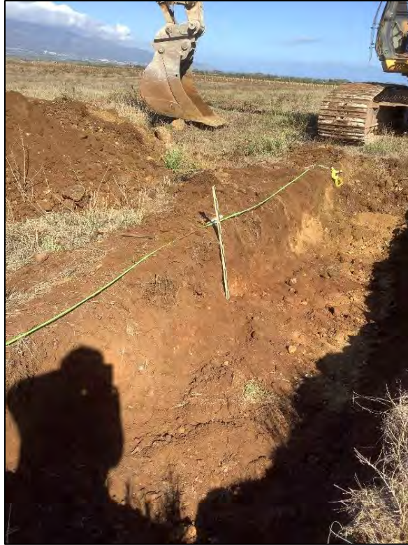
Figure 28. TE-3, general view of west wall, view to northwest
