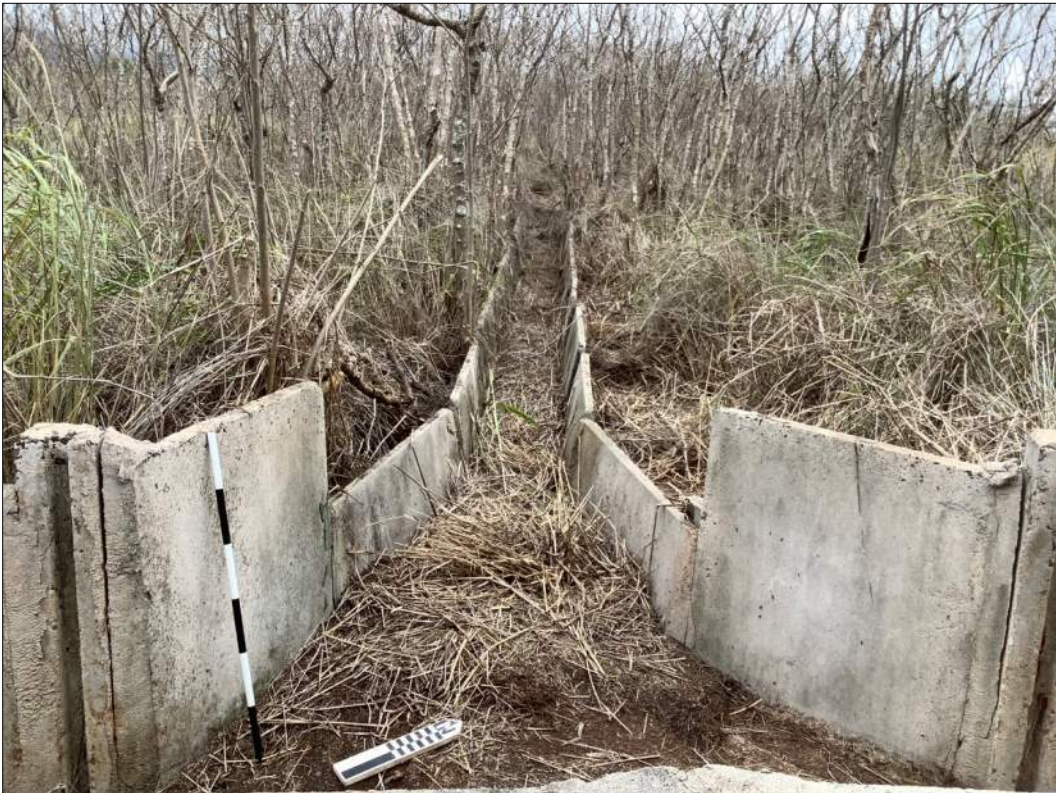
Figure 46. Site 7346 Feature 155-B, view to the northeast from the sluice at the intersection with Site 7346 Feature 155-A.
