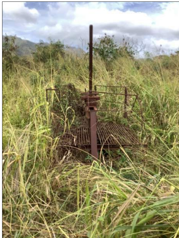
Figure 84. Site 7436 Feature 161-A sluice apparatus.
