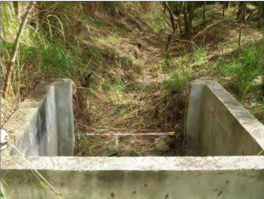
Figure 80. Site 7346 concrete outlet and earthen ditch recorded by Monahan and Thurman (2017:246).
