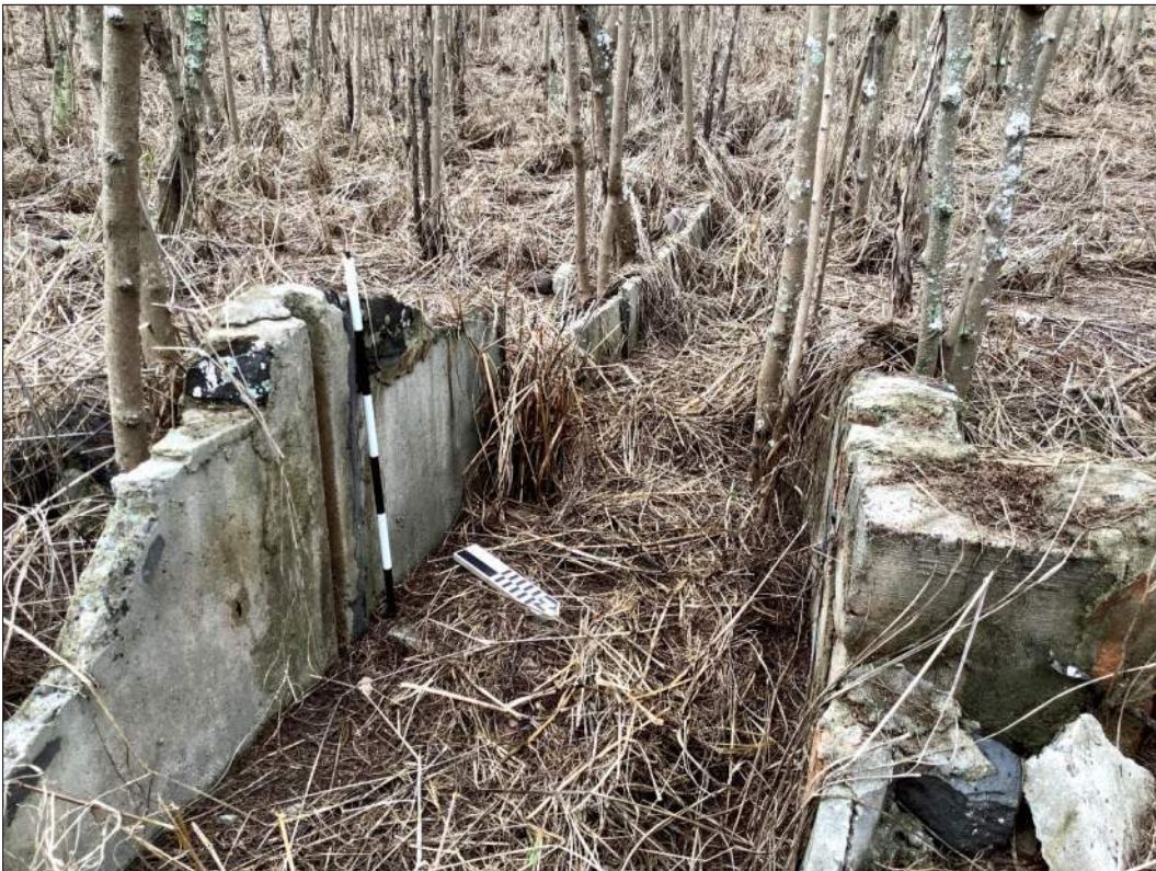
Figure 64. Site 7346 Feature 155-L, former sluice gate location, view to the southwest.
