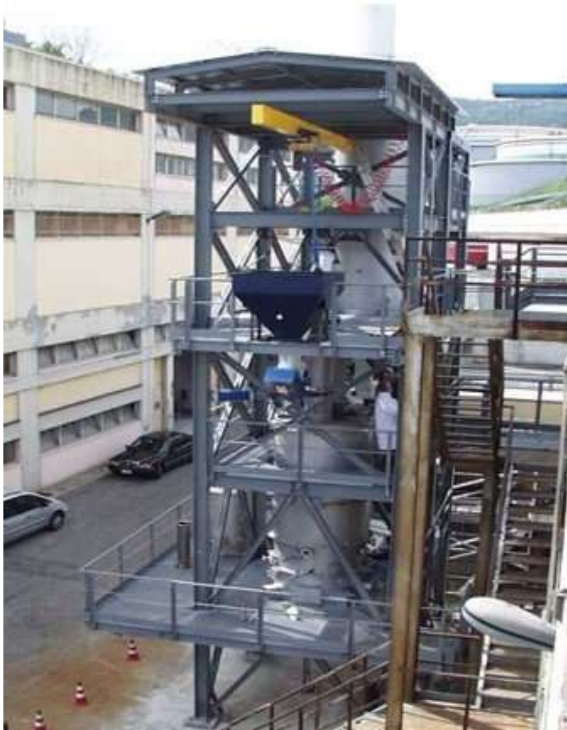
Source: www.energy.gov ; Modular Gasification Test Apparatus at the University of Alaska-Fairbanks
