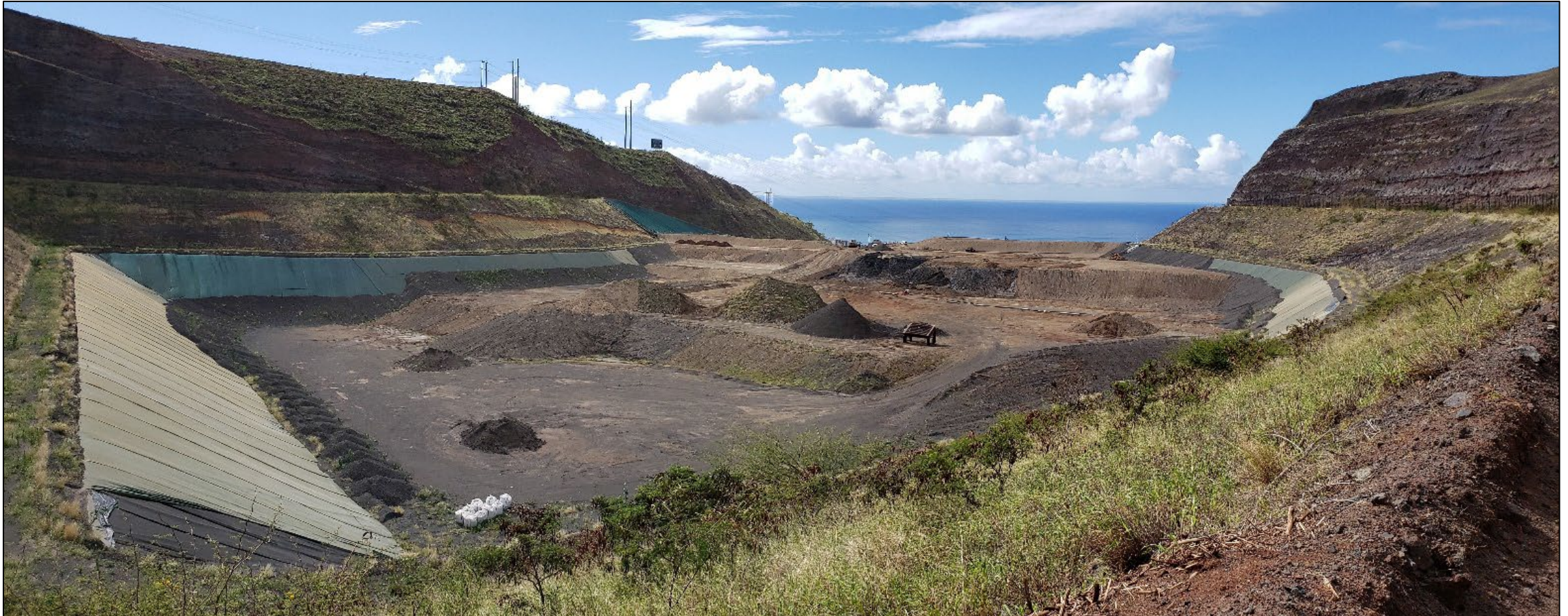
Active ash and municipal solid waste subareas of the Waimanalo Gulch Sanitary Landfill (2022)
