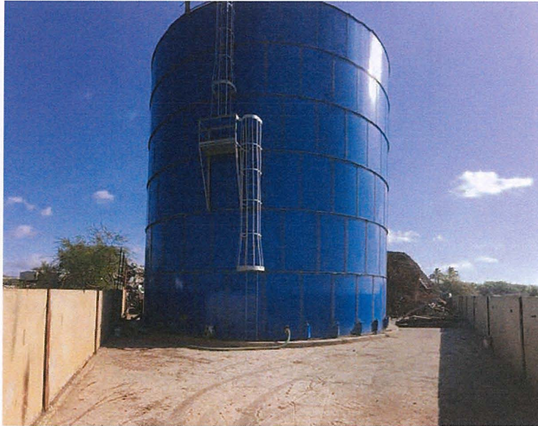
500,000-gallon water tank located on the southwest side of the facility
