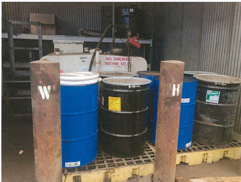
55-gallon drums and AST of hazardous and non-hazardous waste located on secondary spill pallets under covered shed on the northern side of the subject property
