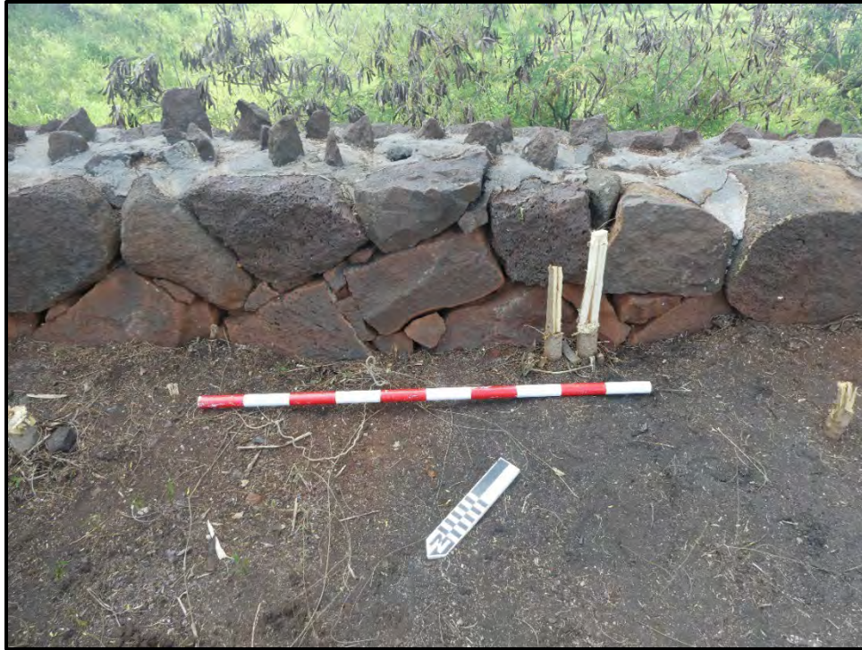
Figure 24. Dam crest detail showing dry-stacked rock wall topped by rock deterrents embedded in mortar; view to the southeast.
