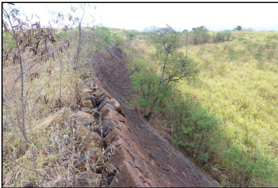
Figure 25. Dam overview showing non-water-facing (south-facing) side; view to the northeast.
