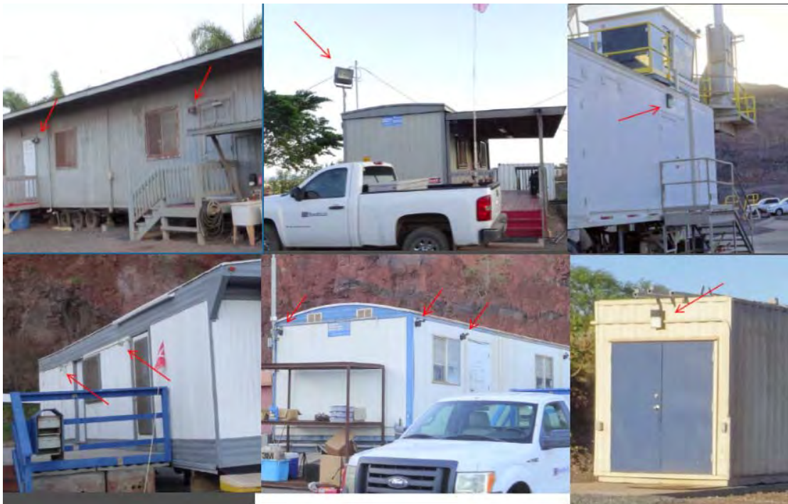
Figure 2 – Quarry - Various light fixtues types. Clockwise from upper left: Office Trailer with wall pack lights; Office Trailer with large floodlight; trailer at Concrete Ready-Mix Plant; Storage Container at Concrete Ready-Mix Plant; Mini floodlights at Maintenance Sheds; and Wall Packs at Maintenance Sheds.
