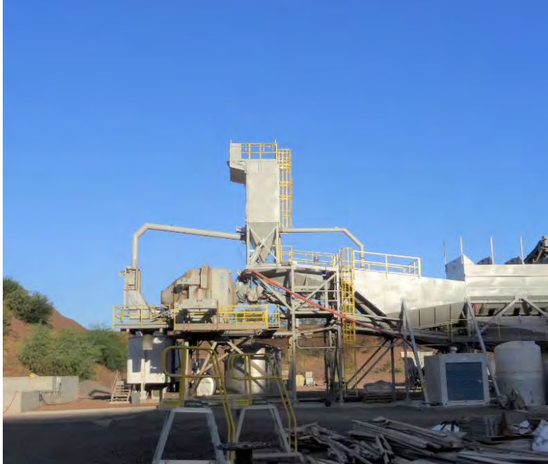
Figure 1 – Concrete Ready-Mix Plant. The tallest part of the sturture appears ideally suited for the mounting of any additional area lighting.
