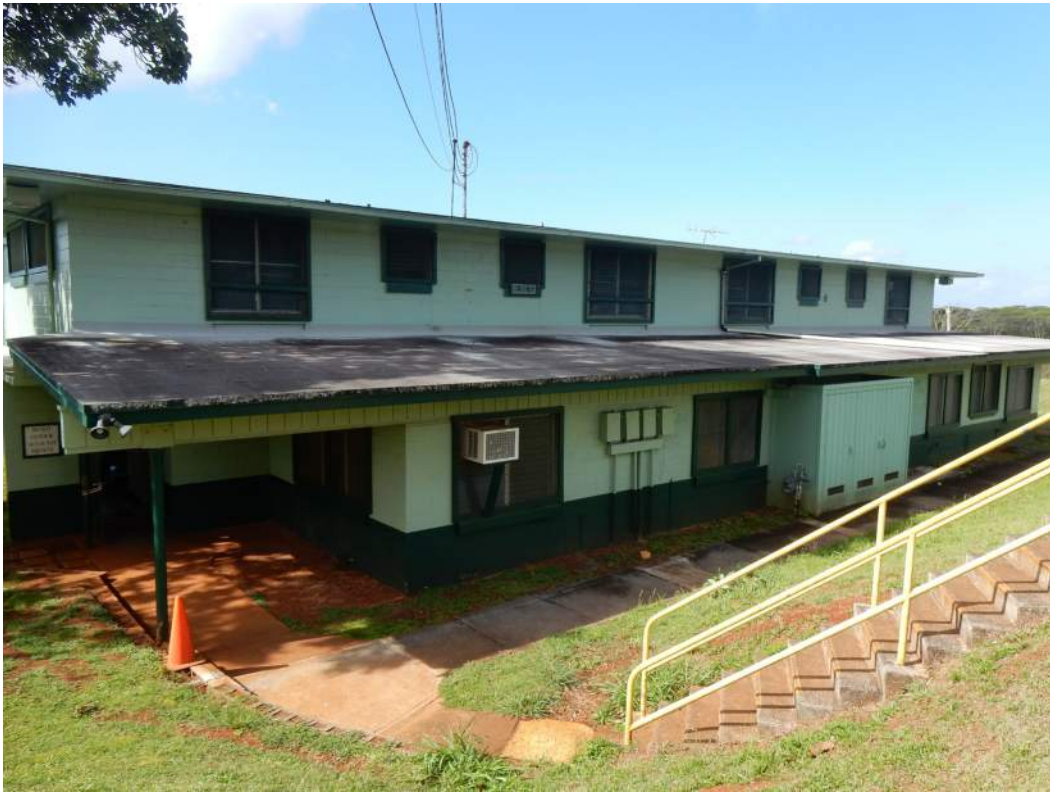
Figure 13: Building 5 North Facade
