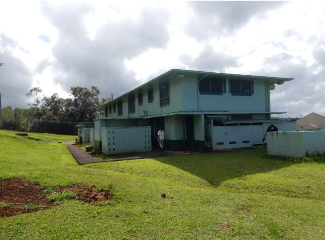
Figure 19: Building 6 West Facade
