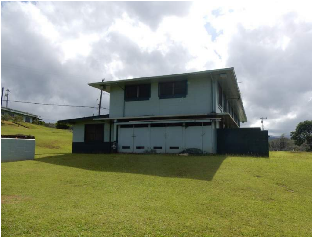
Figure 9: Building 4 West Facade
