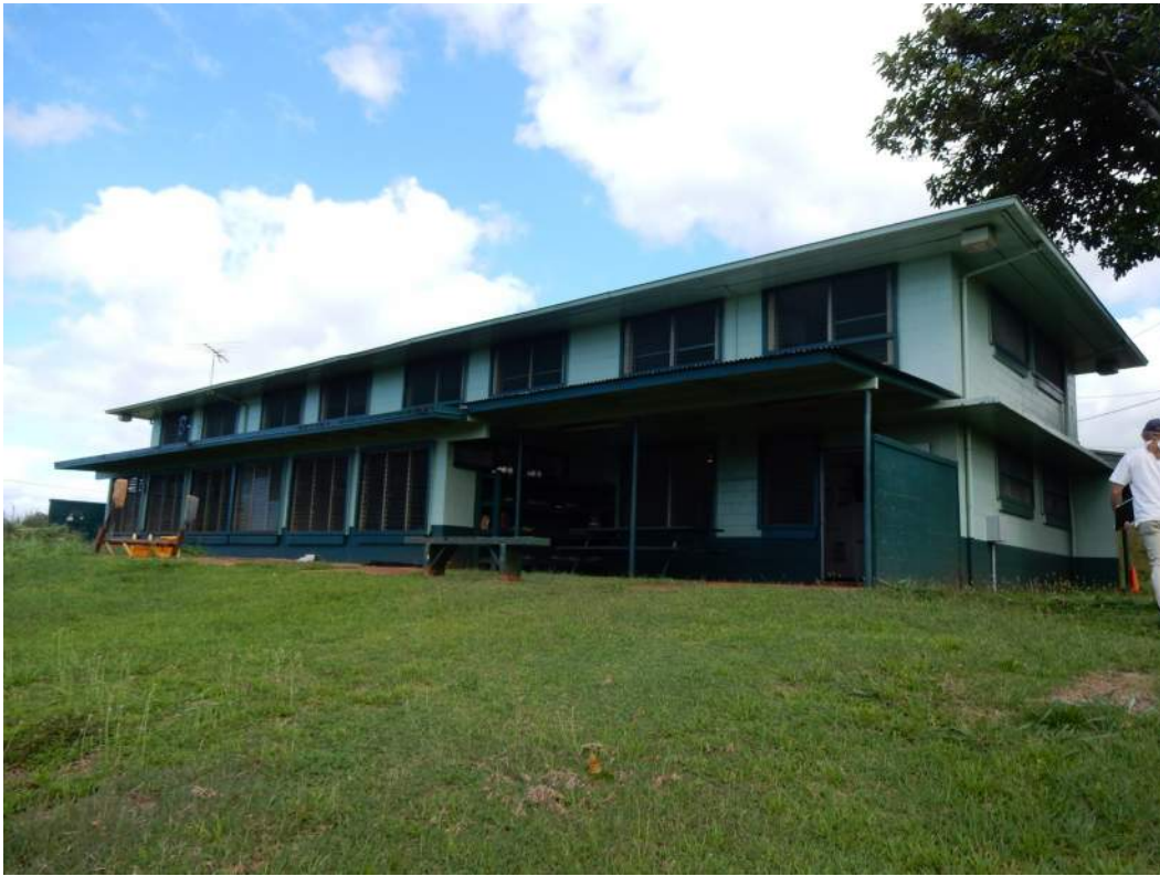
Figure 15: Building 5 South Facade
