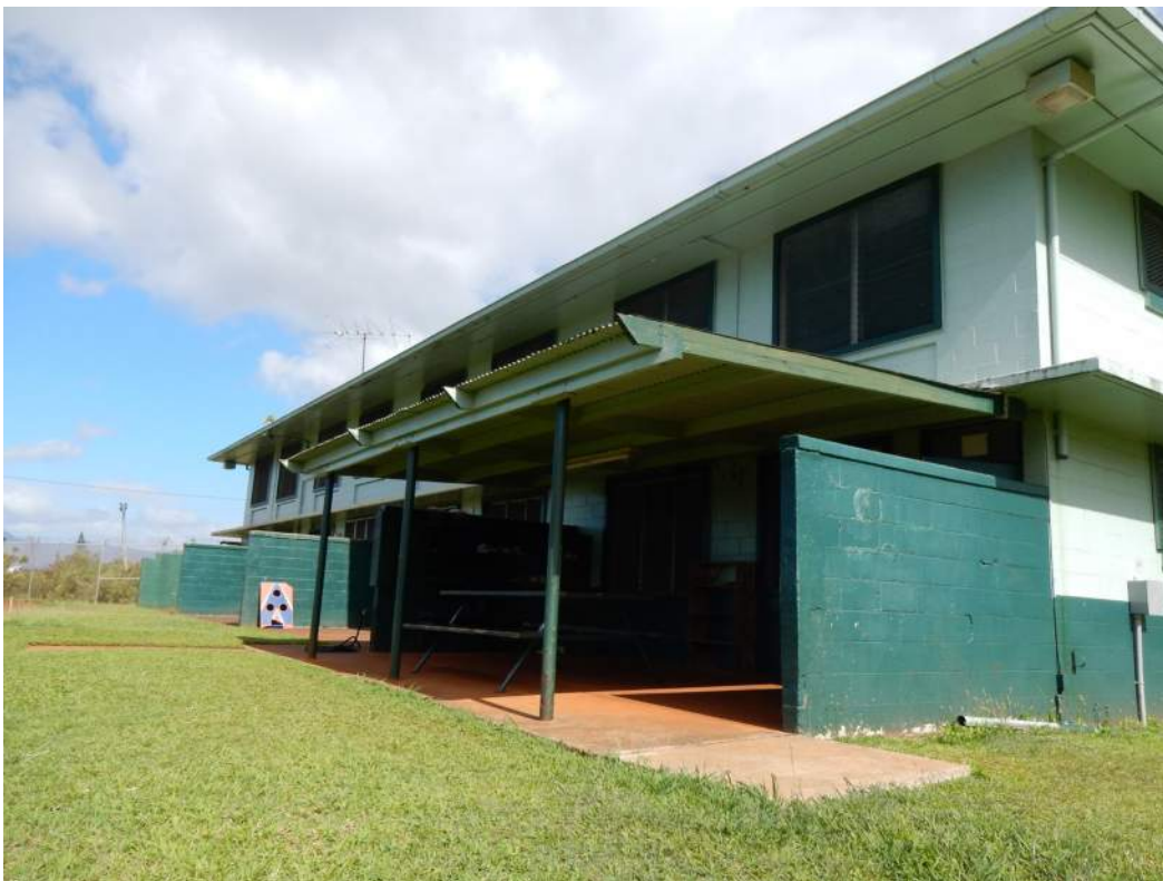
Figure 10: Building 4 South Facade
