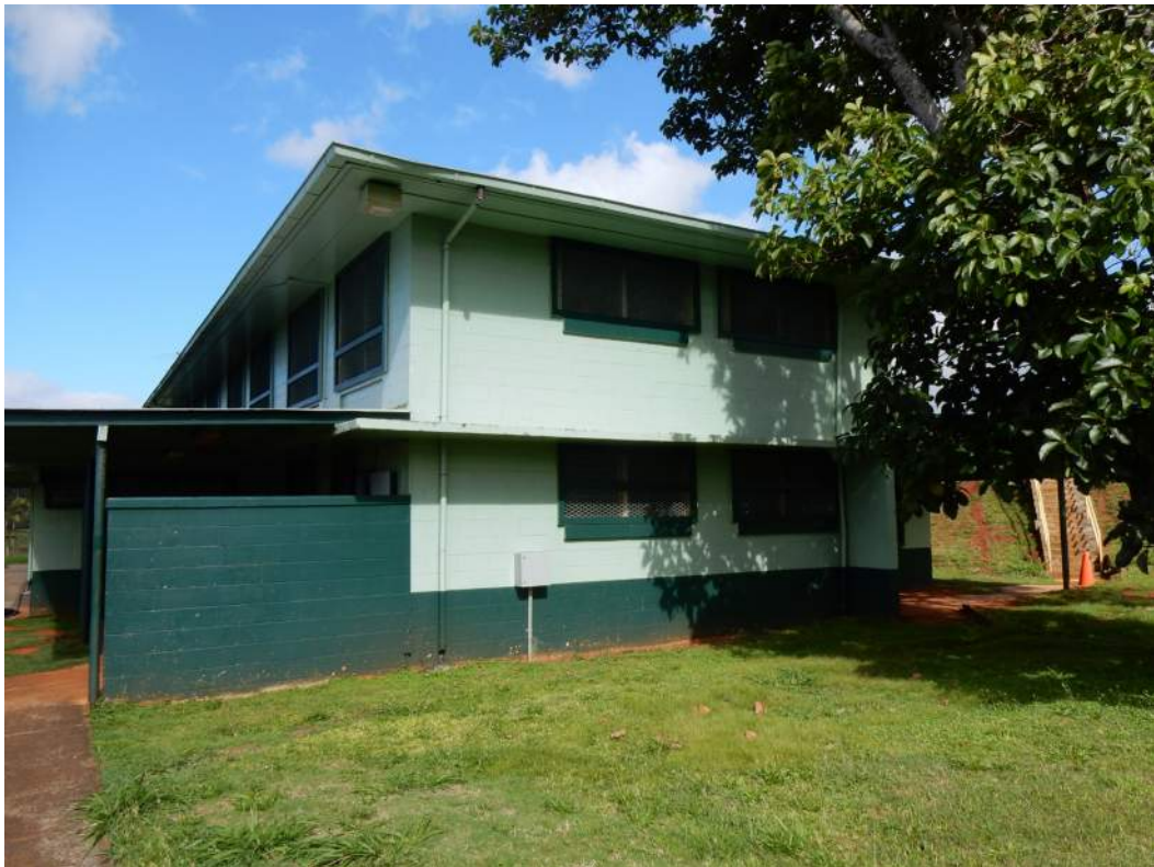
Figure 16: Building 5 East Facade
