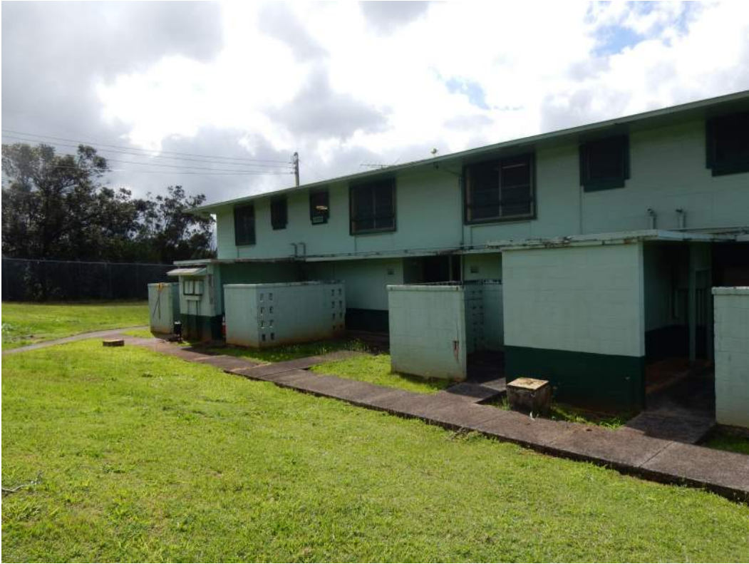
Figure 18: Building 6 North Facade
