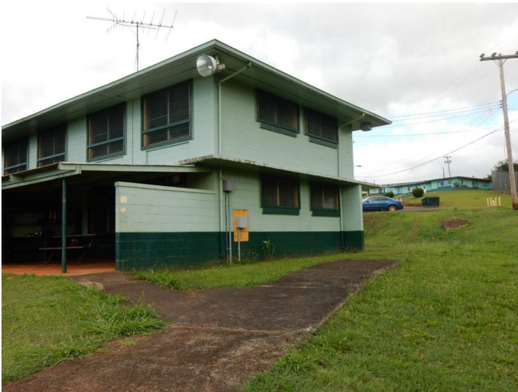
Figure 21: Building 6 East Facade
