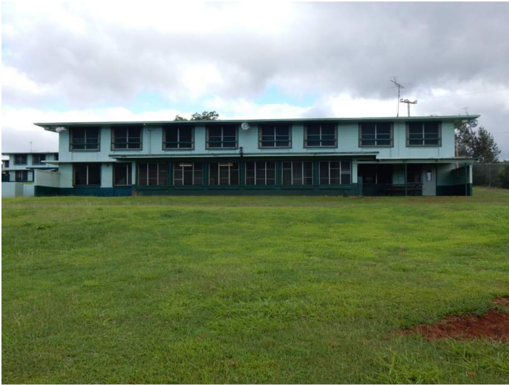
Figure 20: Building 6 South Facade
