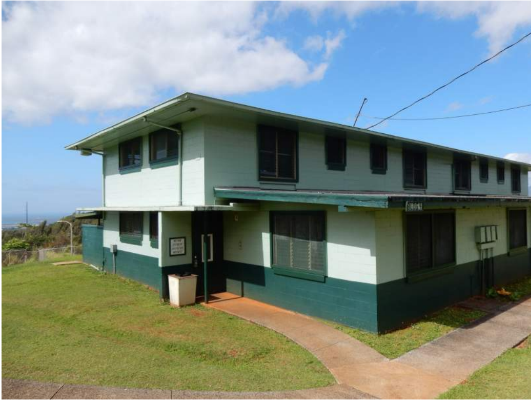
Figure 11: Building 4 East Facade
