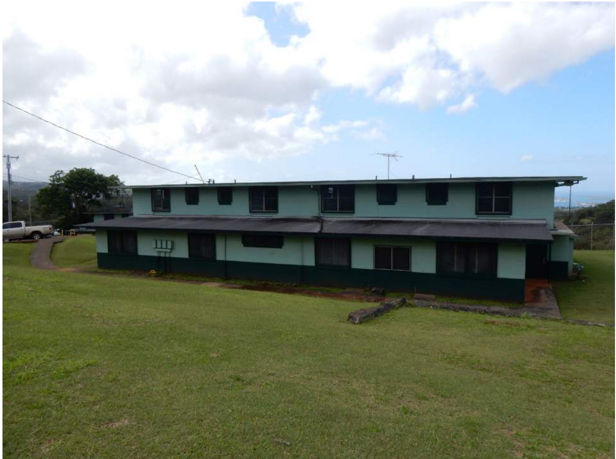
Figure 8: Building 4 North Facade
