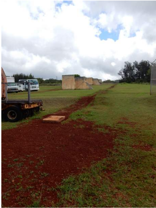
Figure 23: Telecommunication Huts Location
