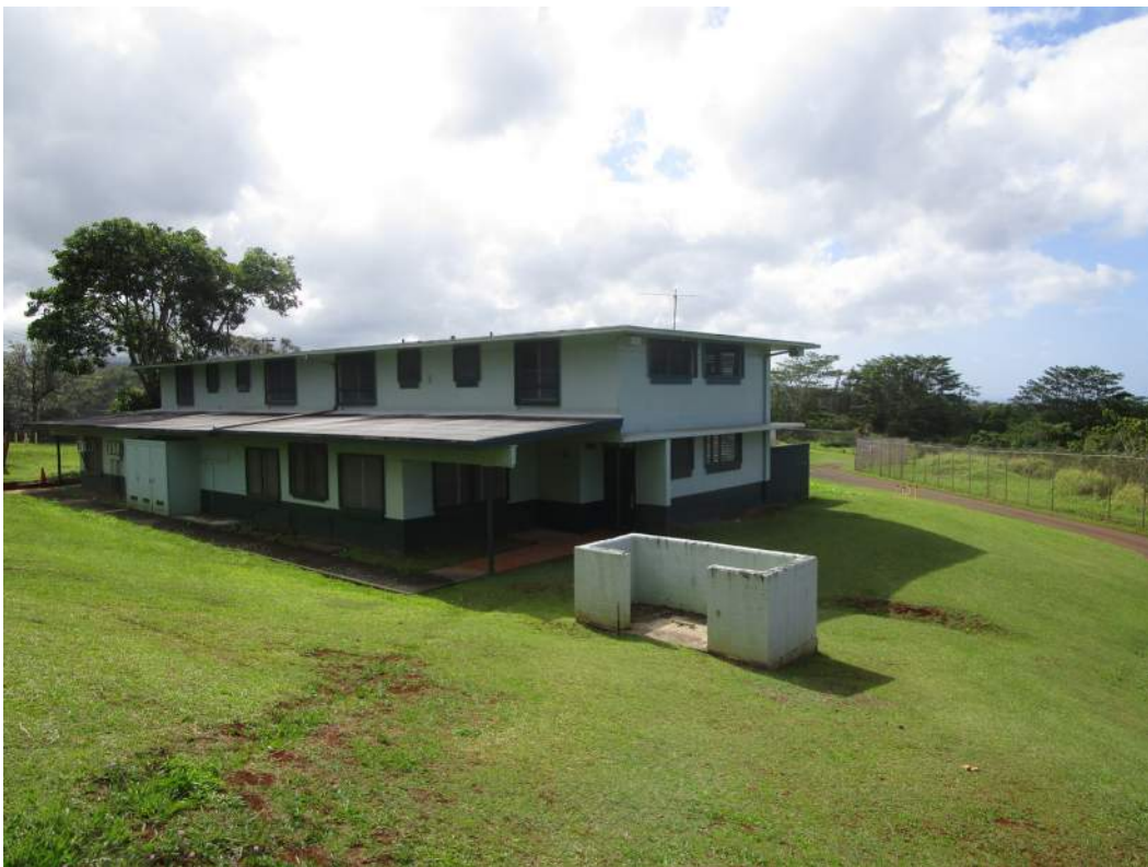
Figure 14: Building 5 West Facade
