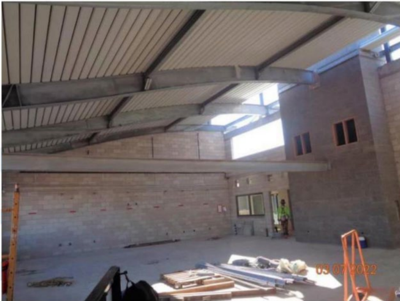
Beams with roof decking on Classroom Building B (Mar. 2022)
