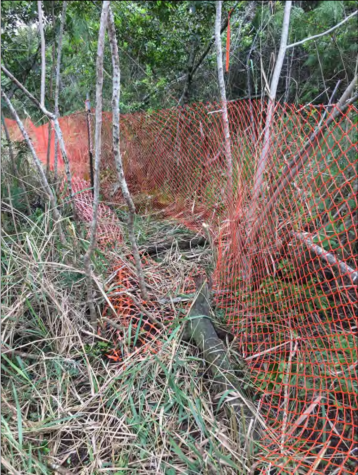
Enclosure 12: Photograph of Site 10736 North Side Construction Buffer Looking East.
