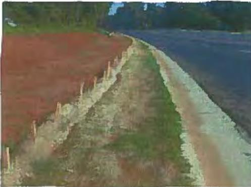
SedimentSTOP consists of a 70% straw / 30% coconut fiber matrix reinforced with a 100% biodegradable netting that is rolled from edge to edge to create a seamless temporary, water-permeable three-dimensional sediment filtration structure.
