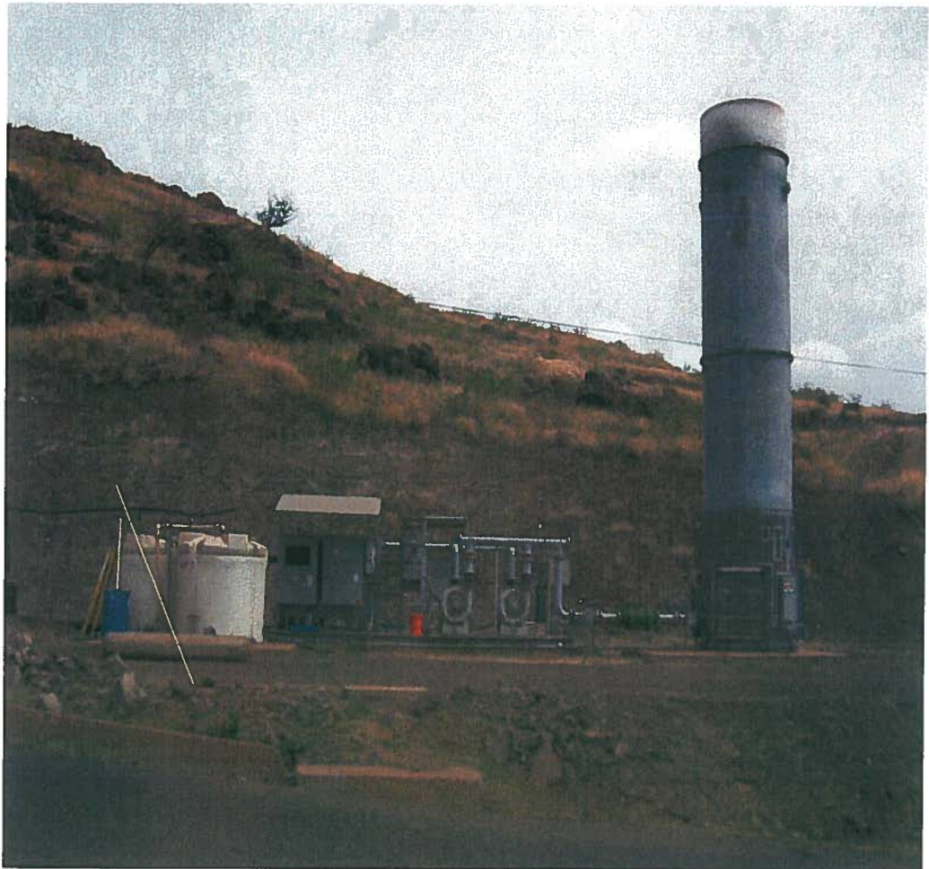
Gas Destruction Flare
