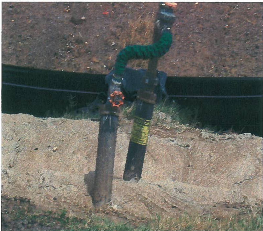
Gas Recovery Well
