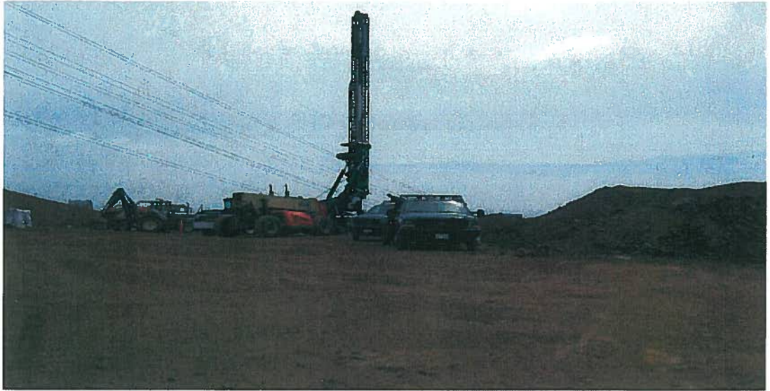
Gas Recovery Well Installation
