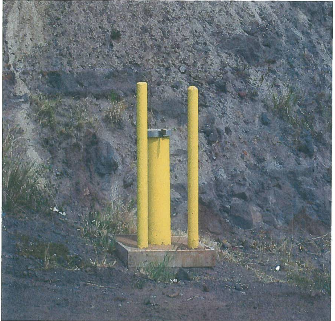
Groundwater Monitoring Well
