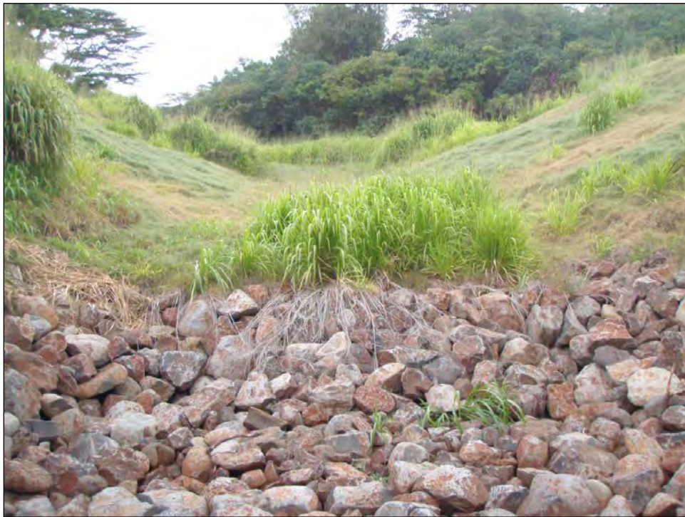
Figure 81. Detail of the recent flood-control alteration of the drainage just below (south of) Reservoir 1-A; Feature 7 (Site 2270) crosses this area from left to right in the background, view north
