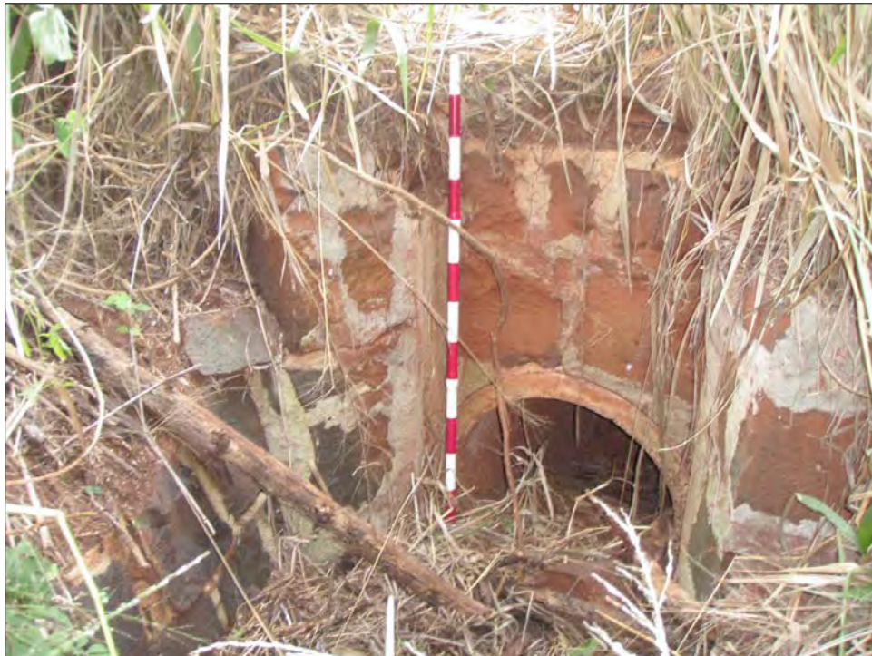
Figure 86. Culvert under earthen road Feature 10, Sub-feature B, Site 2270; view southeast from the north (upslope) side of the road; scale bar is 120 cm high
