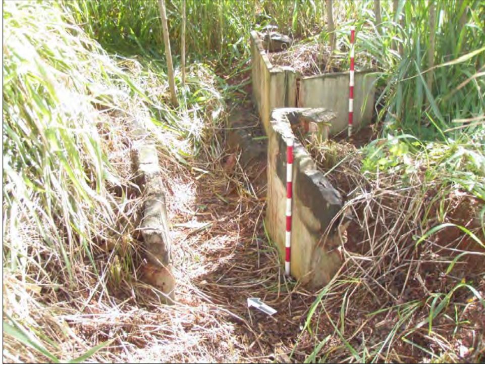
Figure 46. Feature 15, Site 2273, 4-way sluice structure built of both cut basalt and mortar and concrete; view northeast; scale bar in foreground is 80 cm high
