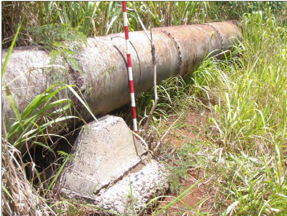
Figure 20. Feature 2, Sub-feature A, Site 2273, showing concrete pad without ferrous-metal brackets, west side of the road, view north-northwest; scale bar marked in 10-cm increments; top of siphon is 90 cm above ground surface
