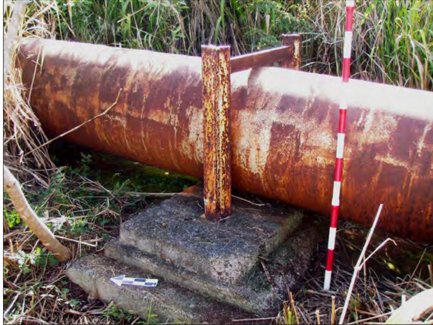
Figure 19. Feature 2, Sub-feature A, Site 2273, showing concrete pad and metal brackets, east side of road, view east; scale bar marked in 10-cm increments; top of siphon is 90 cm above ground surface
