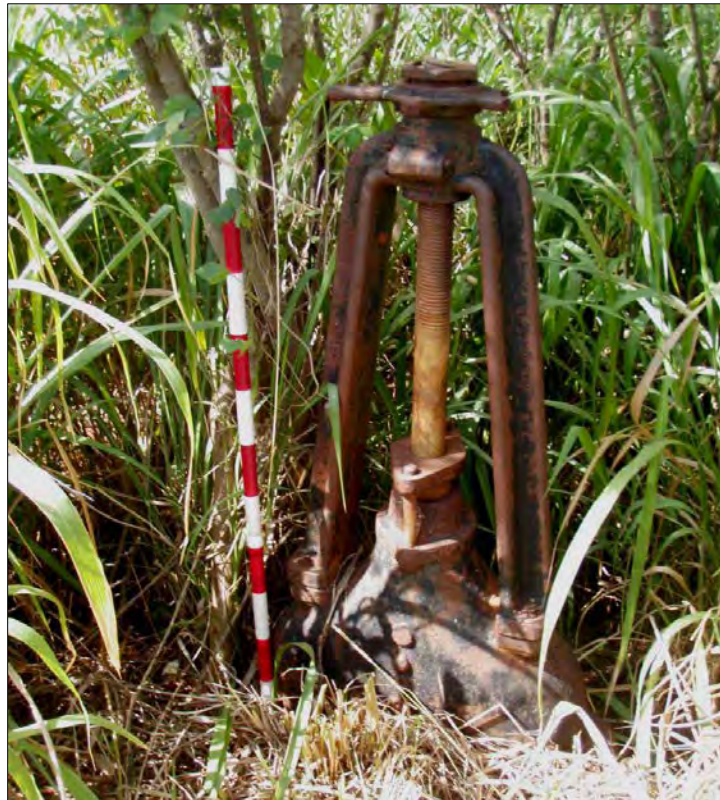
Figure 30. Destroyed hand-operated valve at the intersection of Feature 8 (Site 2273) and Feature 3 (Site 2273), view southeast; scale bar is 120 cm high
