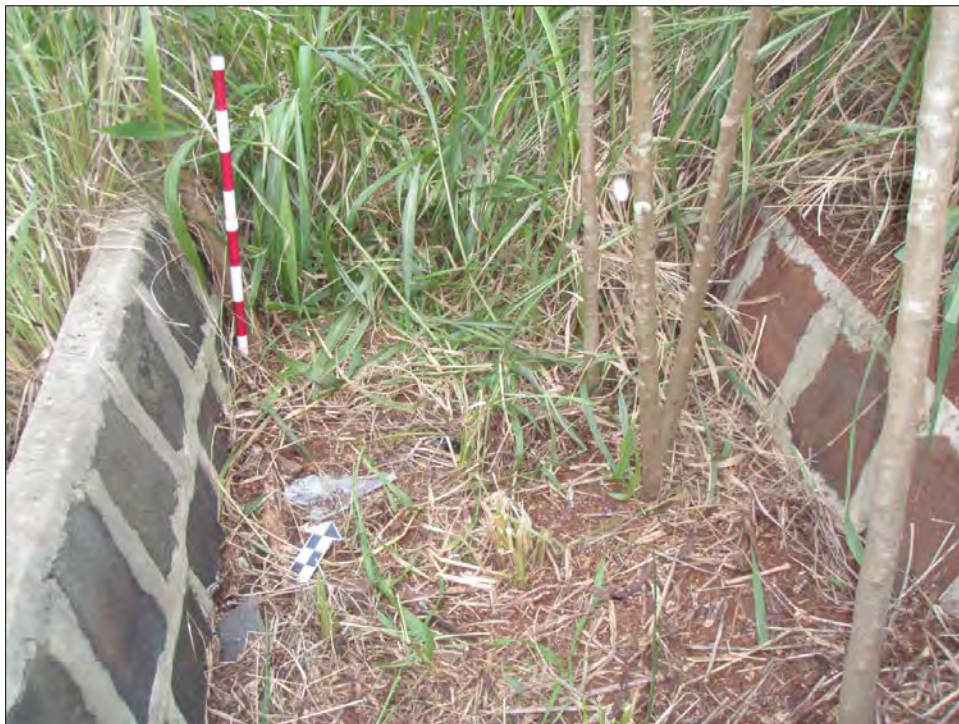
Figure 28. Representative section of cross-slope cut basalt and mortar ditch, Feature 8, Site 2273; view north; vertical scale bar in the base of the ditch is 80 cm long
