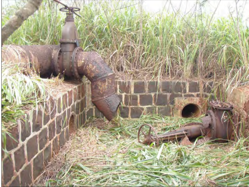
Figure 16. Main basin at Feature 1, Site 2273, showing large hand-operated valves (intact at left, ruined at right); view southwest; basalt and mortar walls are 107-108 cm high
