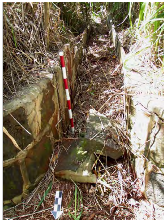
Figure 38. Feature 13, Sub-feature C, Site 2273, view south; sluice gate grooves are in front of scale bar; scale bar is 80 cm high; note, prefabricated concrete flume in background
