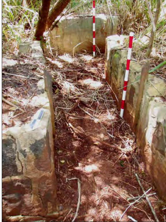
Figure 39. Feature 13, Sub-feature D, Site 2273, view south; sluice gate grooves are in front of the foreground scale bar; cut basalt and mortar opening leads into a short deflection wall/ T-shaped intersection (background); scale bars are 80 cm high
