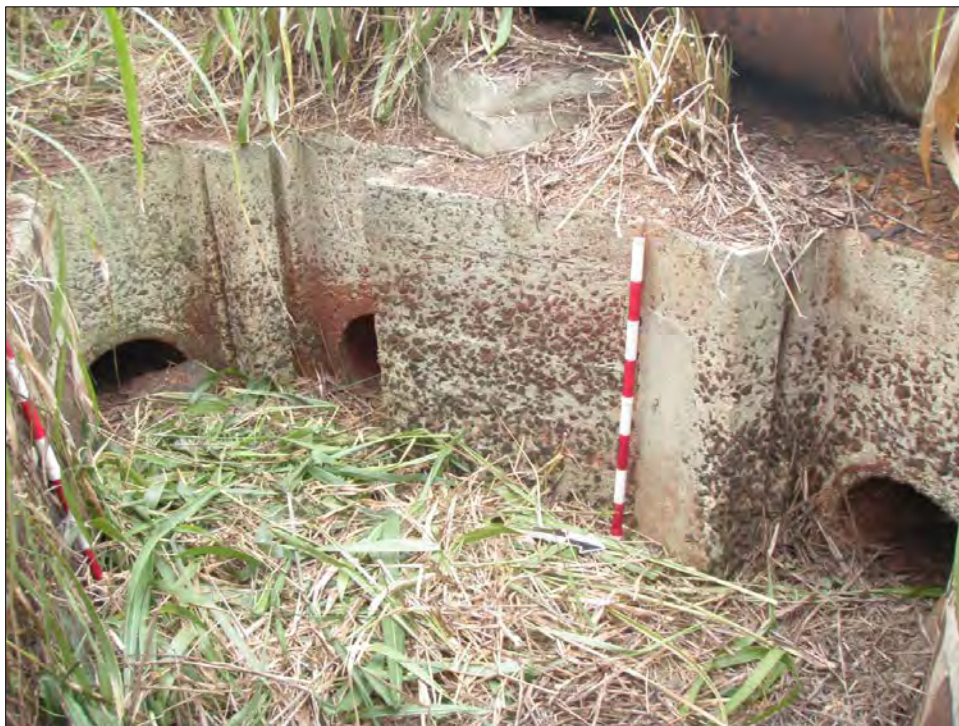
Figure 17. Smaller water-distribution basin, east side of Feature 1, Site 2273; view west-southwest; scale bar to the right is 80 cm high; portion of siphon (Feature 2, Site 2273) is visible at top of image
