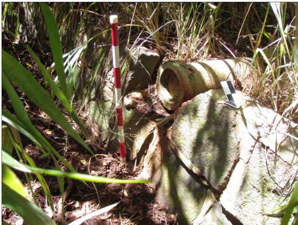
Figure 40. Feature 13, Sub-feature E, Site 2273, view south; concrete pipe with a sheet metal sluice gate through its end, placed into opening along the top of ditch; scale bar is 80 cm high
