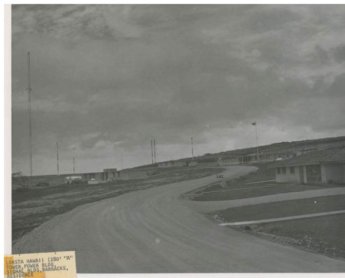
Photo of Newly Graded Road
