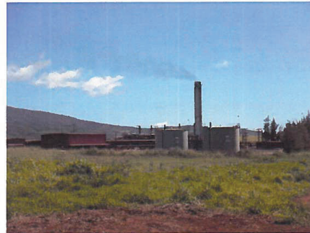
16. MECO power plant facility adjoining the Site.
