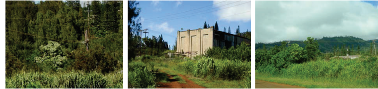
Photos 38-40. Ironwood trees, Kukui nut tree, Lāna'i's old Power Plant and deteriorating house in project area.
