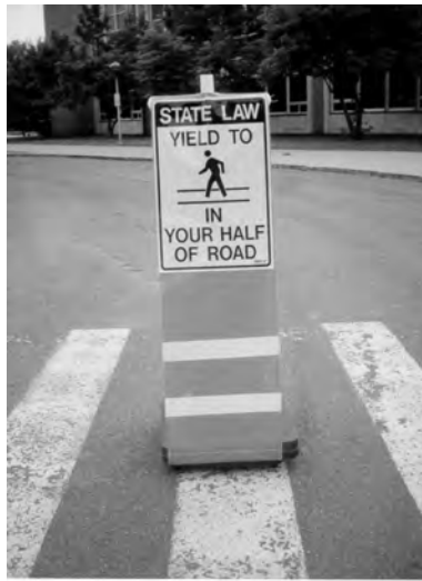
Figure 20. Supplemental Pedestrian Crossing Channelizing Device used in New York State.
