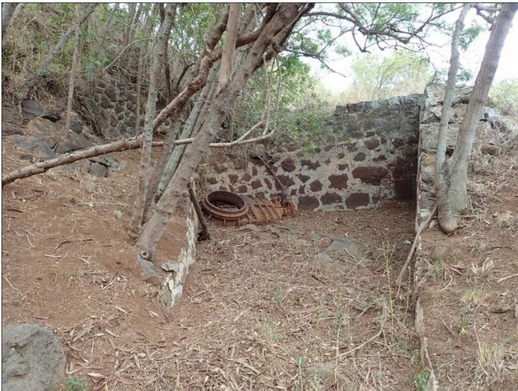
Figure 7. Example of CRM construction.
