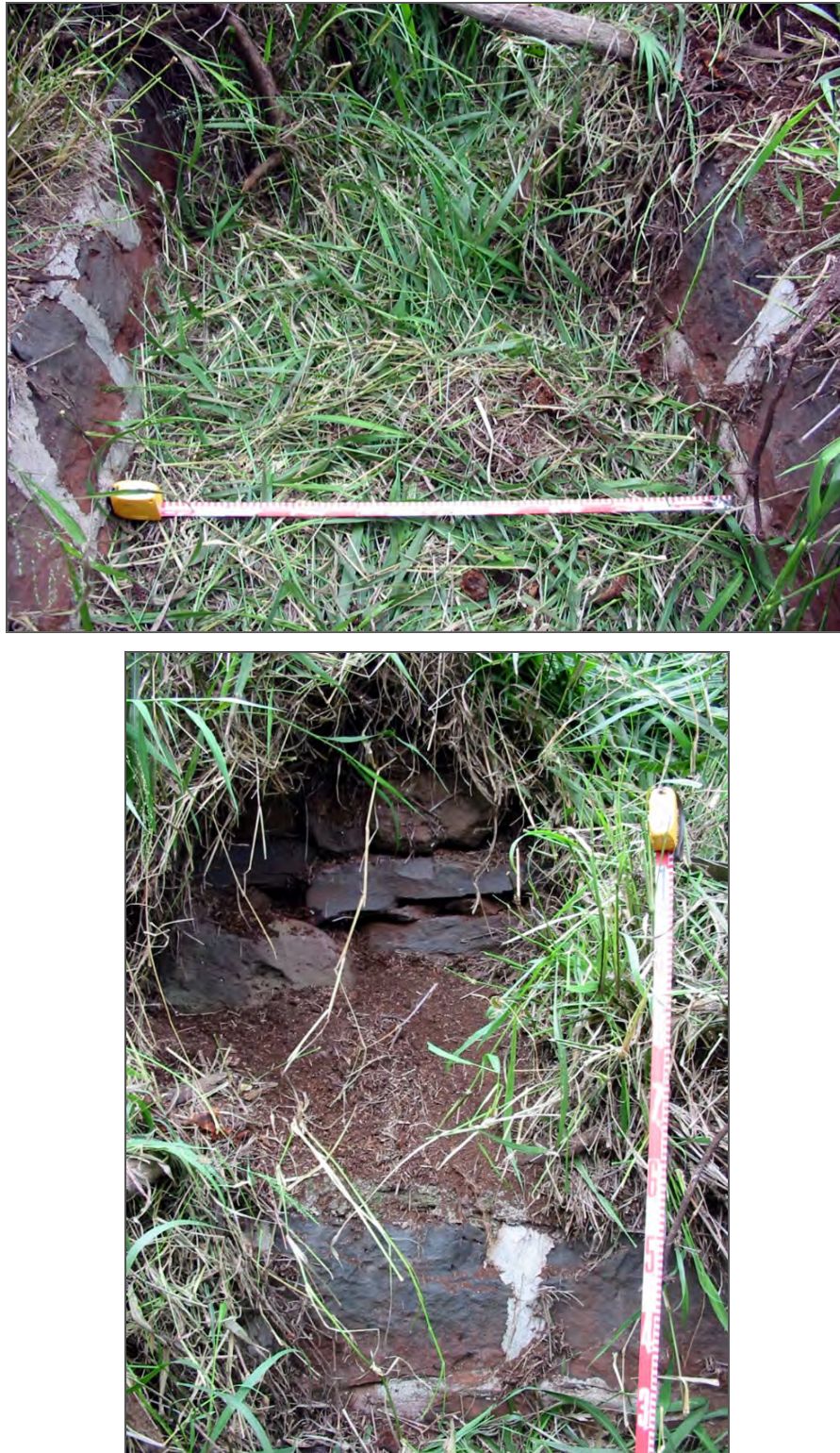
Figure 82. SIHP # 50-80-09-2268 showing the dressed basalt boulder and mortar Waiahole Ditch (top), and stacked basalt boulder and cobble retaining wall (below) (Tulchin and Hammatt 2004:53)
