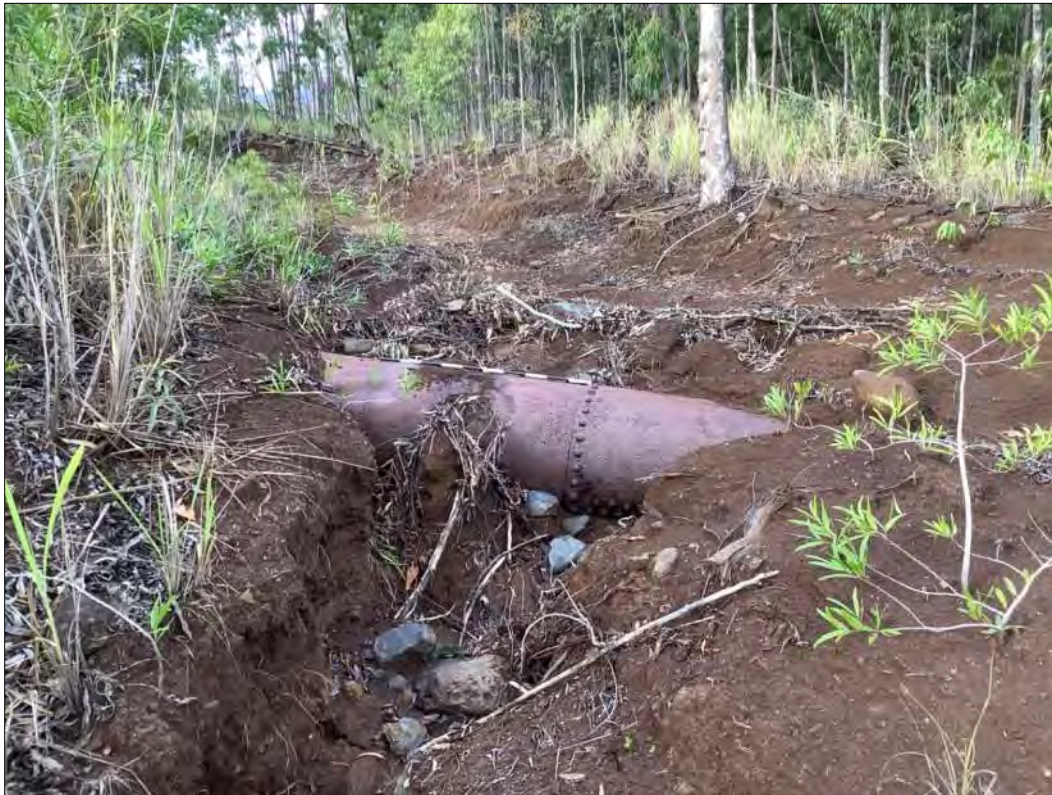
Figure 82. Exposed metal aqueduct pipe.
