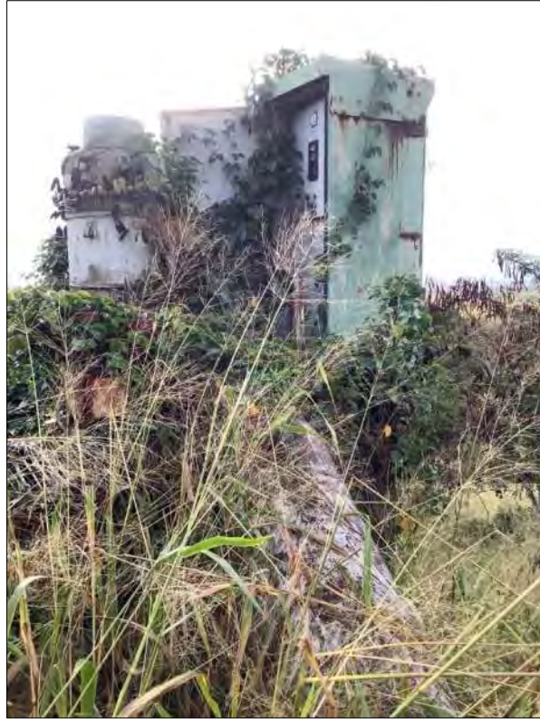
Figure 83. Pump house and siphon.
