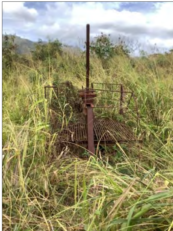
Figure 84. Site 7436 Feature 161-A sluice apparatus.
