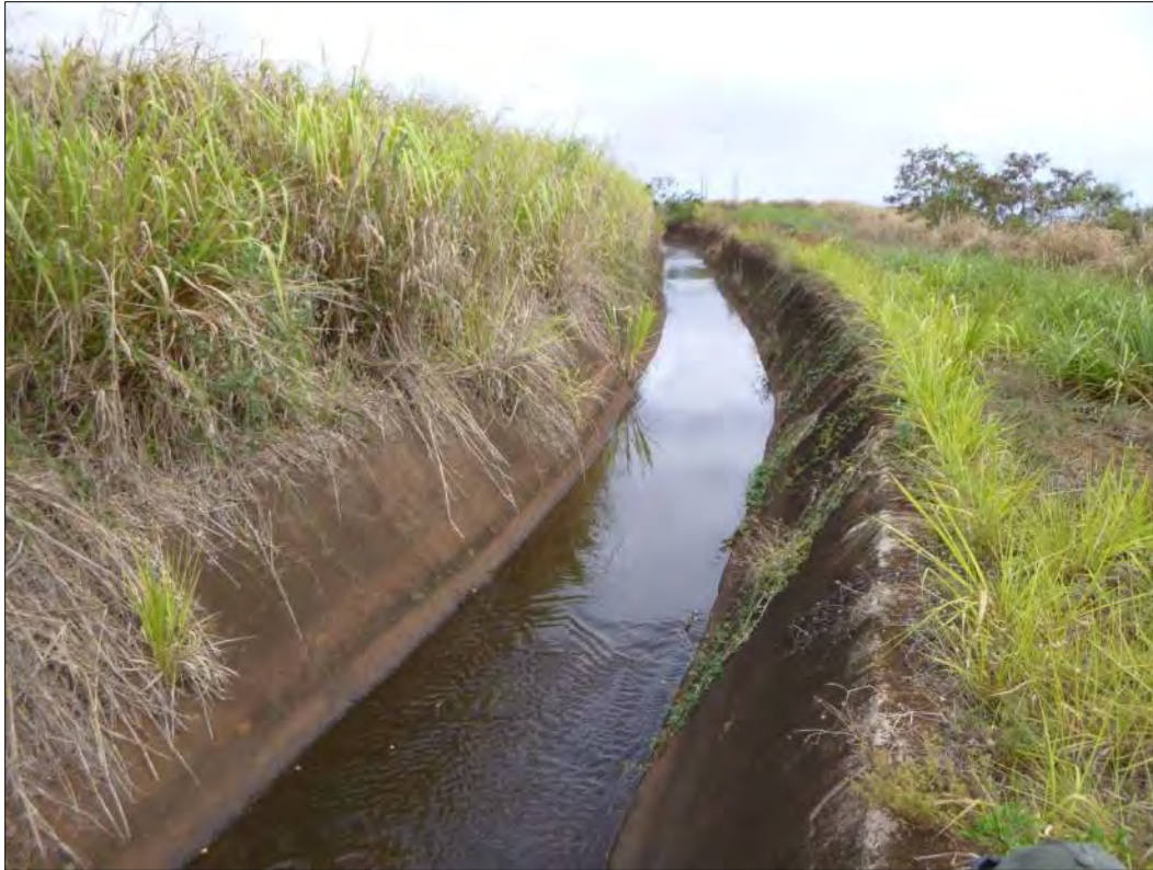
Figure 41. 1916 concreted section of the Waiāhole Ditch.
