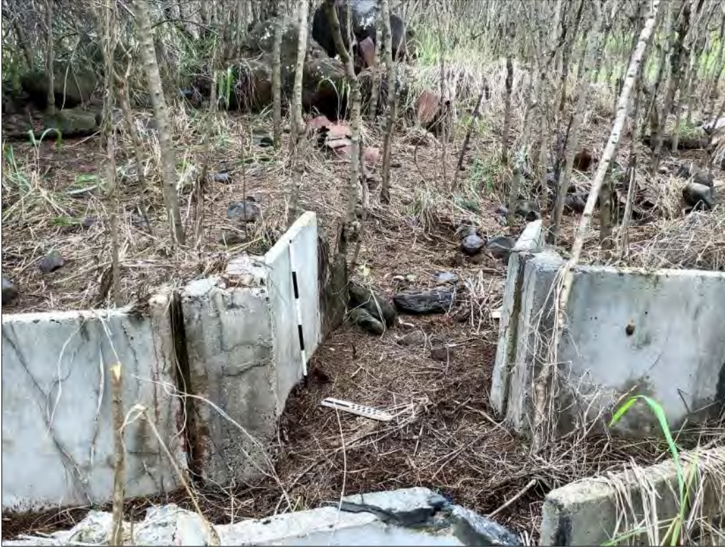
Figure 70. Site 7346 Feature 155-M, sluice gate indicating the presence of a former western flume branch at the northern end of the southernmost section, view to the southwest.
