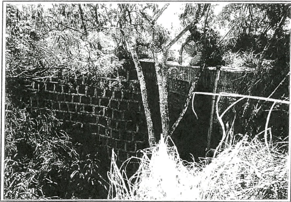
Figure 6: Irrigation System Bridge. Note Date of 1928 in Center of Bridge. View to Southeast.
