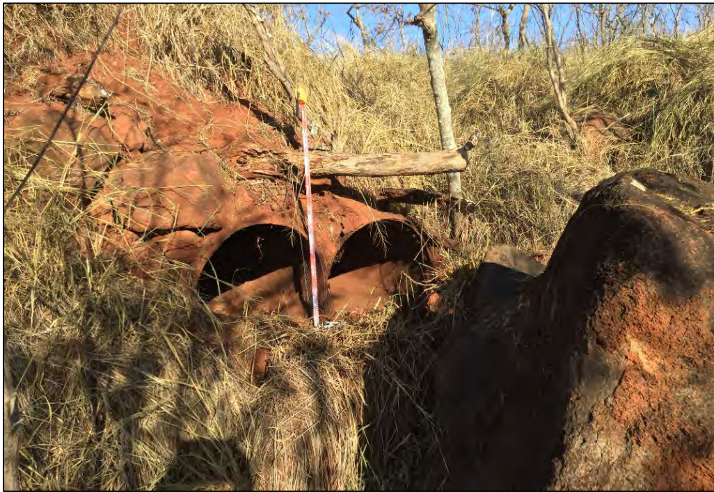
Figure 49. Lower portion of SIHP # 50-80-08-5593 Feature 1 showing metal pipes, view to northwest
