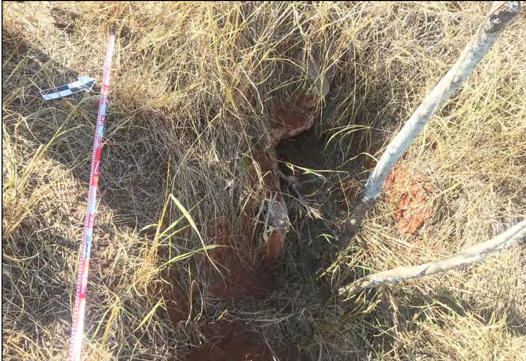
Figure 77. SIHP # 50-80-08-5593 Feature 2E, culvert remnants, view to northwest
