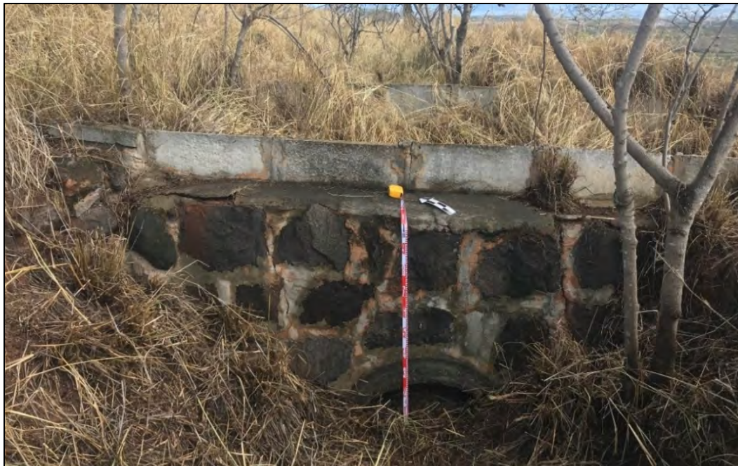
Figure 102. SIHP # 50-80-09-2268 Feature E, culvert and bridge components of the Waiahole Ditch in southern project area, view to northeast
