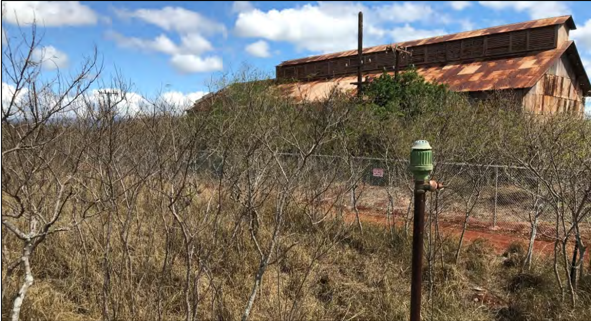
Figure 46. Mill building immediately southeast of the project area boundary (downslope of Feature 2A complex), view to east
