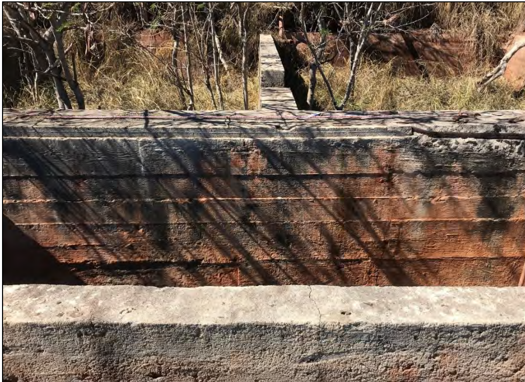
Figure 64. Overview of SIHP # 50-80-08-5593 Feature 2B, showing two large water storage compartments (background) and smaller compartment containing pipes and valves (foreground), view to northwest
