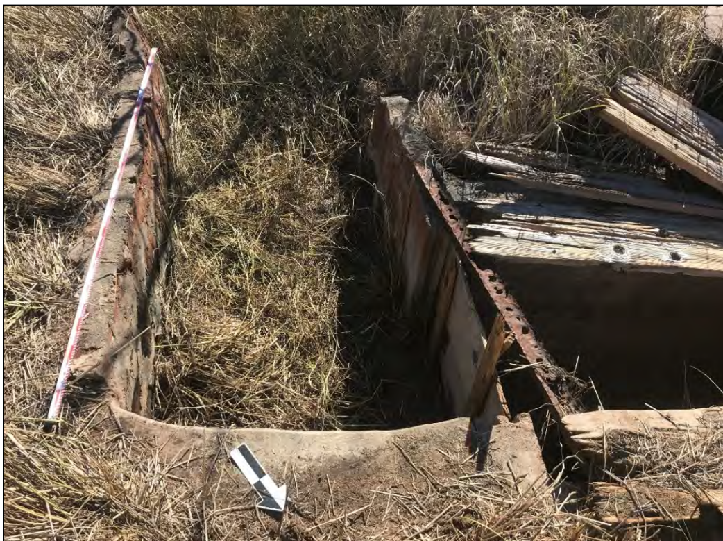
Figure 75. Feature 2D plan view of southern retention area with sluice gate and possible overflow channel, view to southwest
