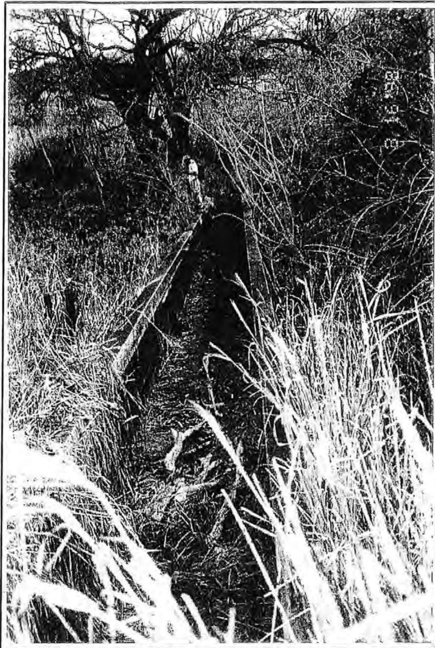
Figure 7: Site 2268, a Section of Water Flume. View to Northeast.
