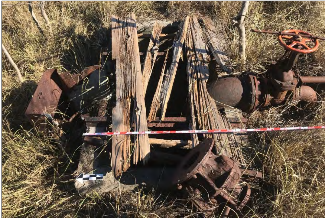
Figure 72. Overview of SIHP # 50-80-08-5593 Feature 2D, northeast valve box, view to east
