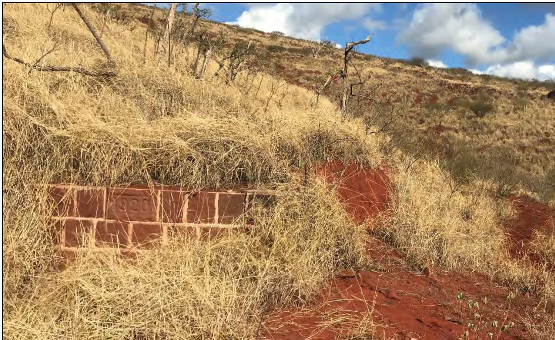
Figure 96. Portion of SIHP # 50-80-09-2268, Waiahole Ditch outside (north) of project area, with date “1920” inscribed on basalt and mortar culvert, view to northeast
