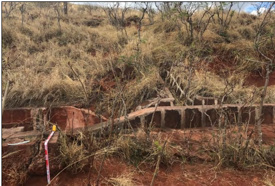
Figure 59. Overview of SIHP # 50-80-08-5593 Feature 2A complex with eastern flume (right), extending into SIHP # 50-80-09-2268 Waiahole Ditch, view to northwest
