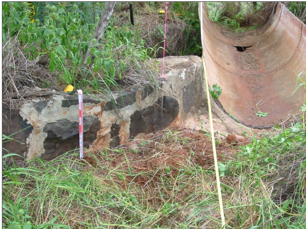
Figure 85. SIHP # 50-80-09-2268 Feature B, showing stone and mortar flume support foundation, view to north (Hunkin and Hammatt 2009:50)
