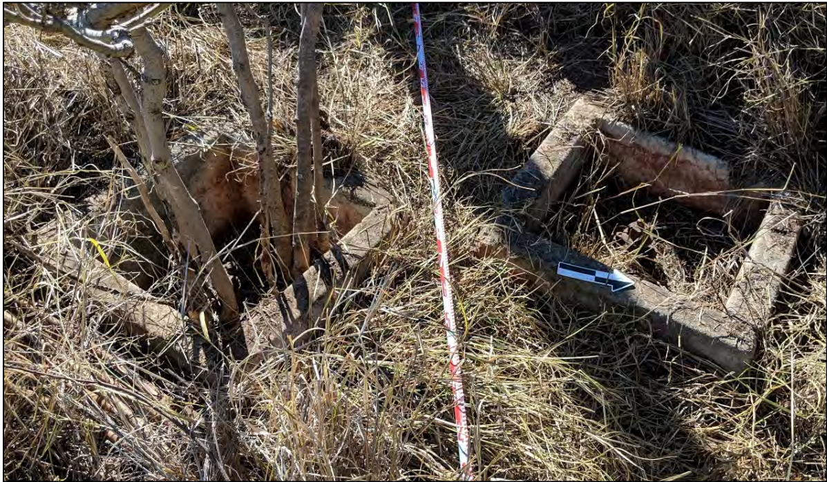
Figure 68. Concrete valve components of SIHP # 50-80-08-5593 Feature 2C, view to west
