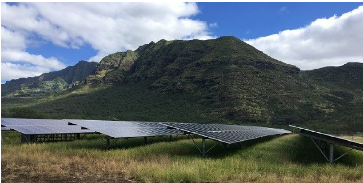
Photograph 2. View of typical solar photovoltaic modules on a fixed-tilt racking system ( O'ahu, Hawai'i )
