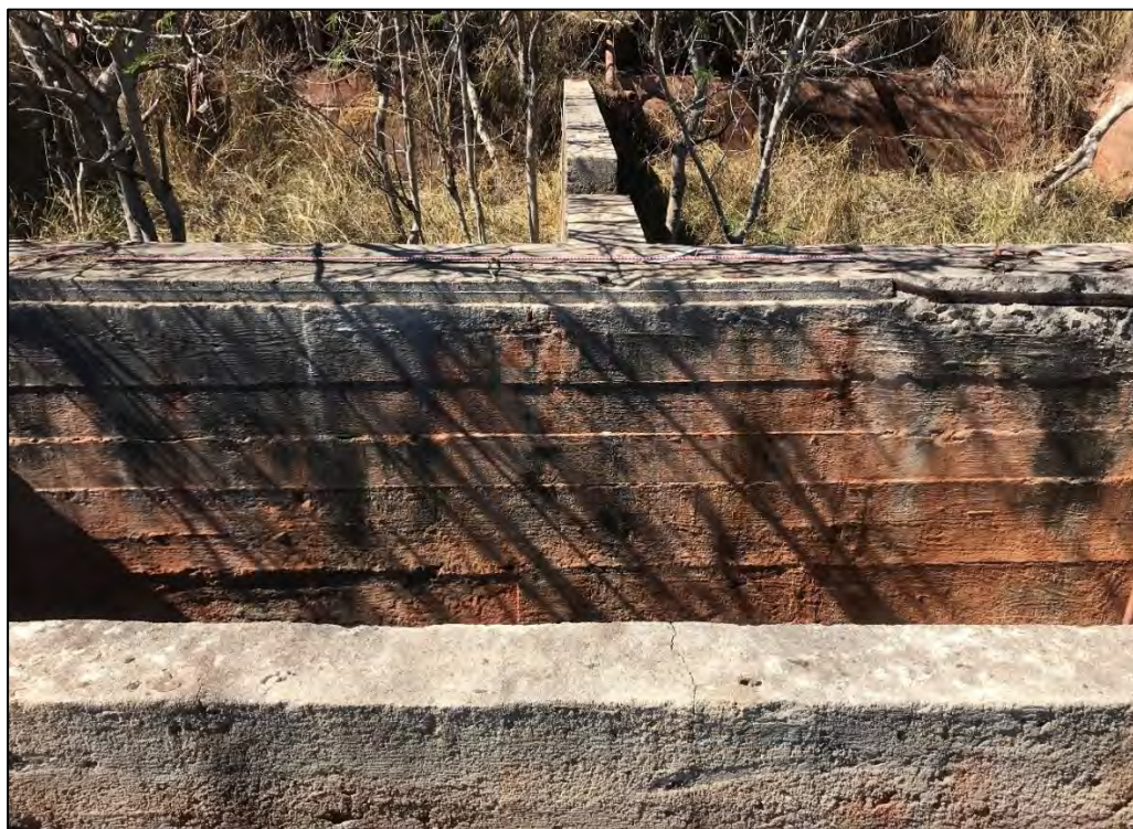
Figure 62. Overview of SIHP # 50-80-08-5593 Feature 2B, showing two large water storage compartments (background) and smaller compartment containing pipes and valves (foreground), view to northwest
