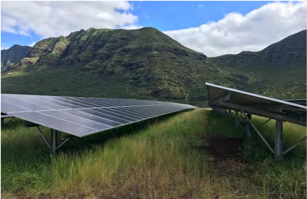
Photograph 1. View of typical solar photovoltaic modules on a fixed-tilt racking system ( O'ahu, Hawai'i )
