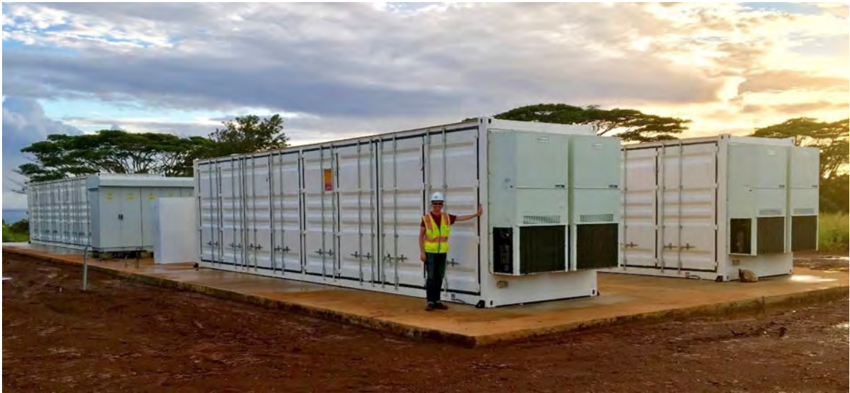
Photograph 3. View of typical battery units and associated equipment on concrete equipment pad ( Kaua'i, Hawai'i )
