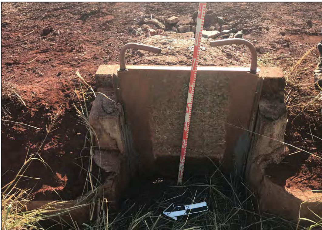
Figure 126. SIHP # 50-80-09-2268 Feature K, showing culvert with intact sluice gate, view to east
