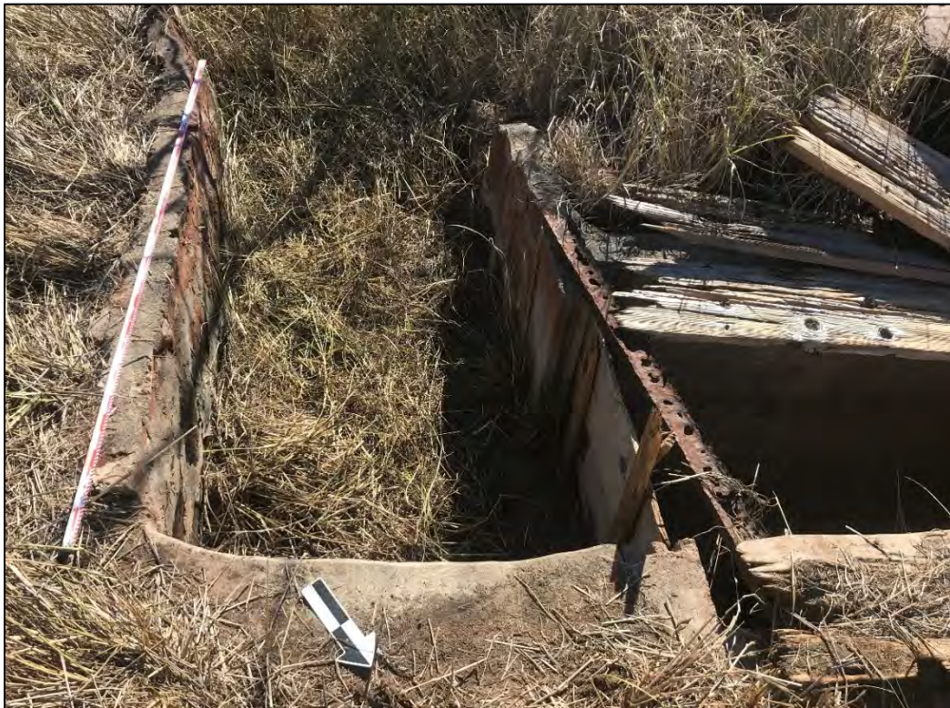
Figure 75. Feature 2D plan view of southern retention area with sluice gate and possible overflow channel, view to southwest
