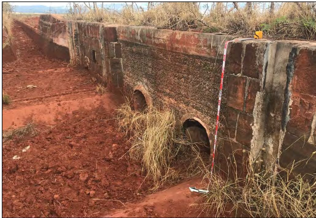
Figure 54. Overview of SIHP # 50-80-08-5593 Feature 2A and SIHP # 50-80-09-2268 Waiahole Ditch portion, with catchment basin (foreground) and drain pipes, view to east
