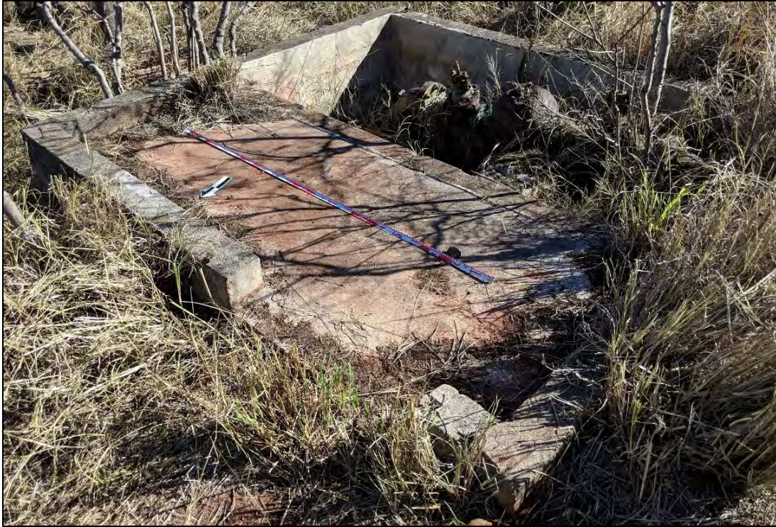
Figure 69. Overview of concrete foundation and pipes component of SIHP # 50-80-08-5593 Feature 2C, view to southeast
