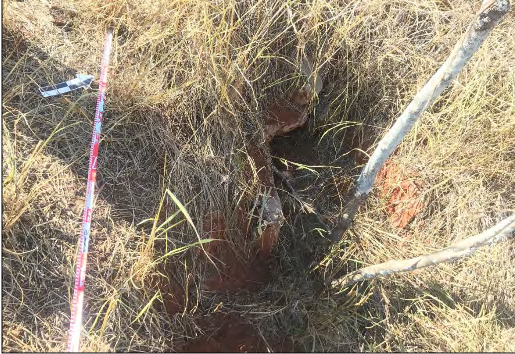
Figure 77. SIHP # 50-80-08-5593 Feature 2E, culvert remnants, view to northwest
