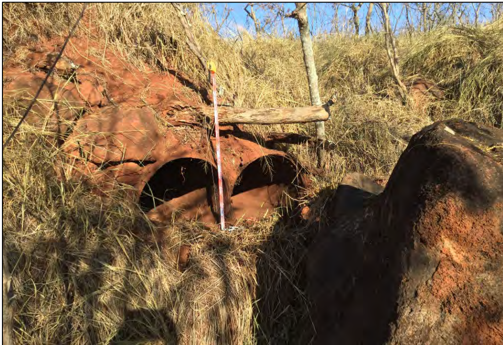
Figure 49. Lower portion of SIHP # 50-80-08-5593 Feature 1 showing metal pipes, view to northwest
