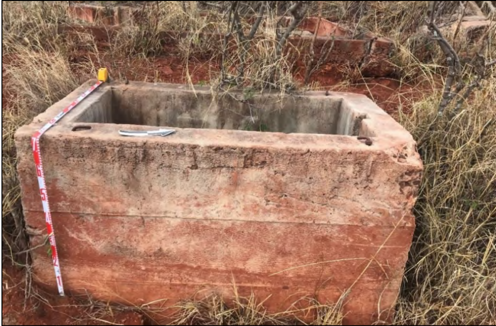
Figure 60. Water retention component of SIHP # 50-80-09-5593 Feature 2A complex, view to west
