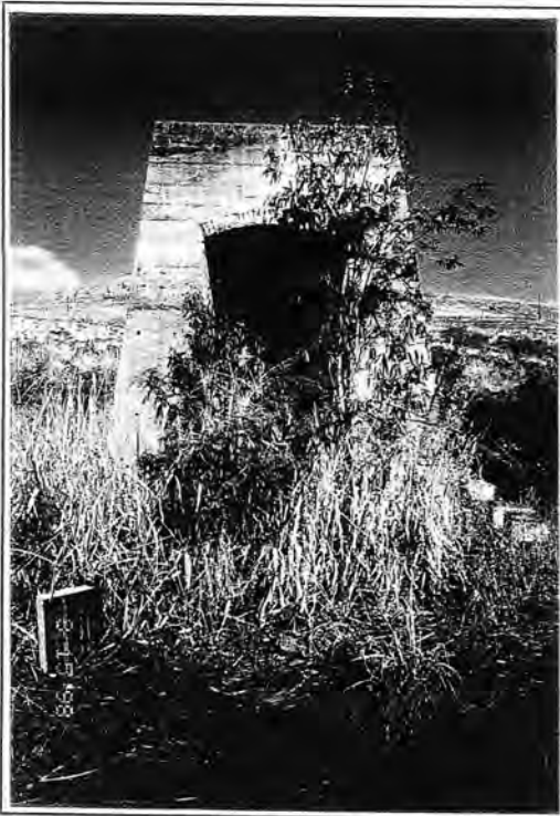
Figure 3: Pump House No. 12. View to Northwest.
