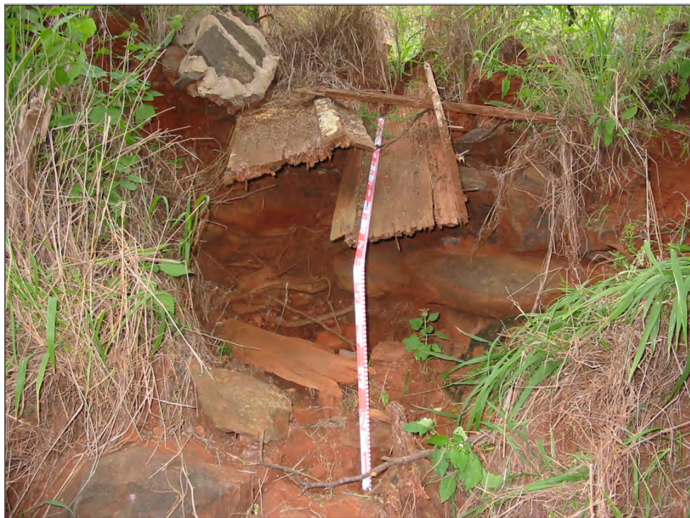
Figure 86. SIHP # 50-80-09-2268 Feature B flume, showing wooden flume extension (Hunkin and Hammatt 2009:50), view to southeast
