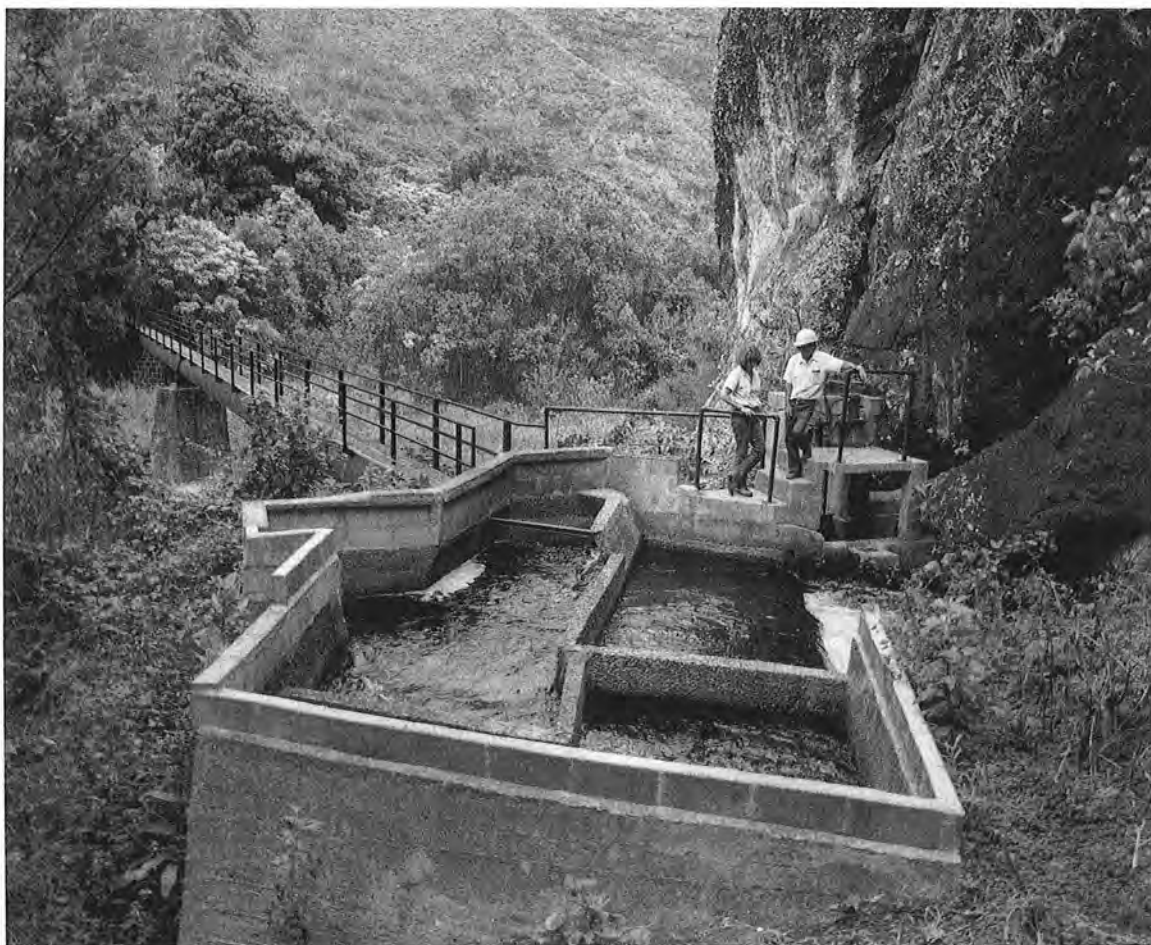
Water is collected in this gravel trap before being sent on its way in the Iao-Maniania Ditch. (Photo: D. Franzen.)
