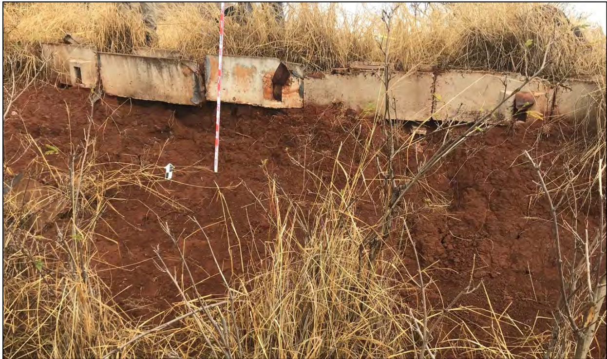
Figure 32. Remnant water diversion flume in southern project area, view to north
