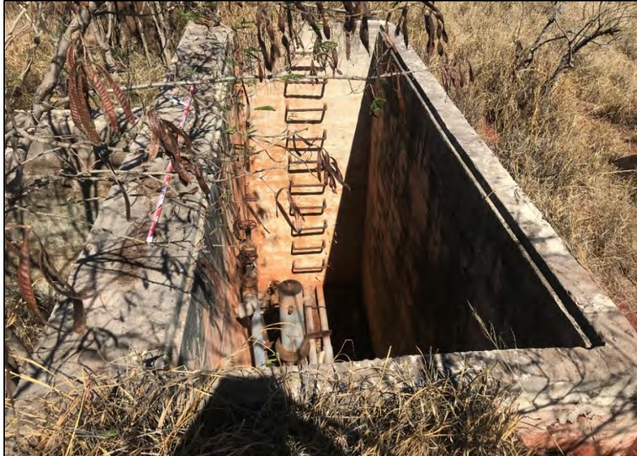
Figure 65. Overview of SIHP # 50-80-08-5593 Feature 2B, smaller southeast portion, view to northeast
