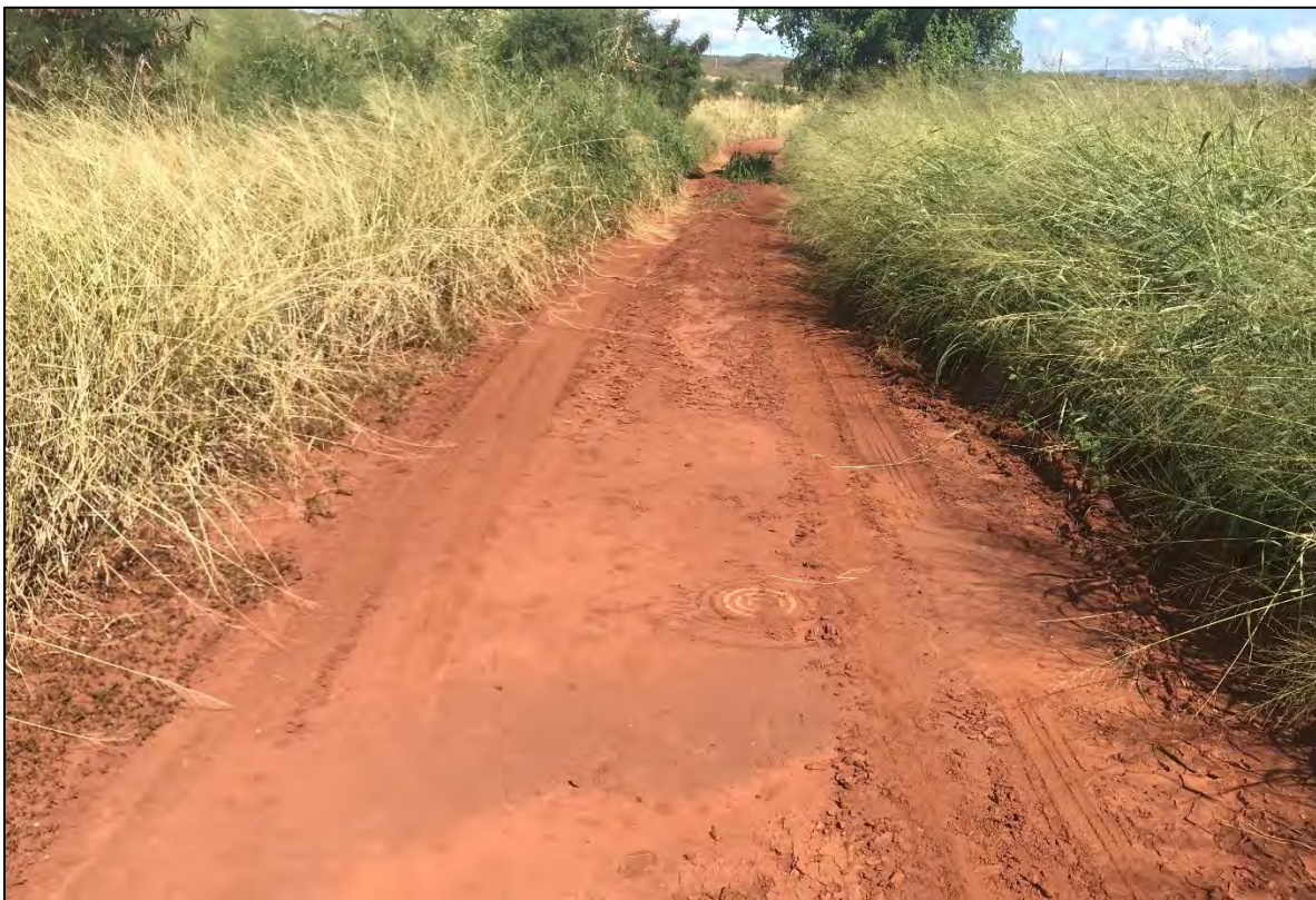
Figure 36. Access road overview showing water manhole, view to northeast
