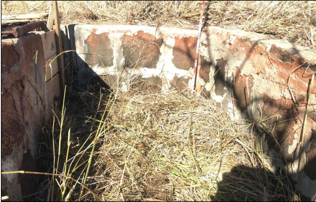
Figure 74. SIHP # 50-80-08-5593 Feature 2D sluice gate and possible water overflow channel, view to northeast
