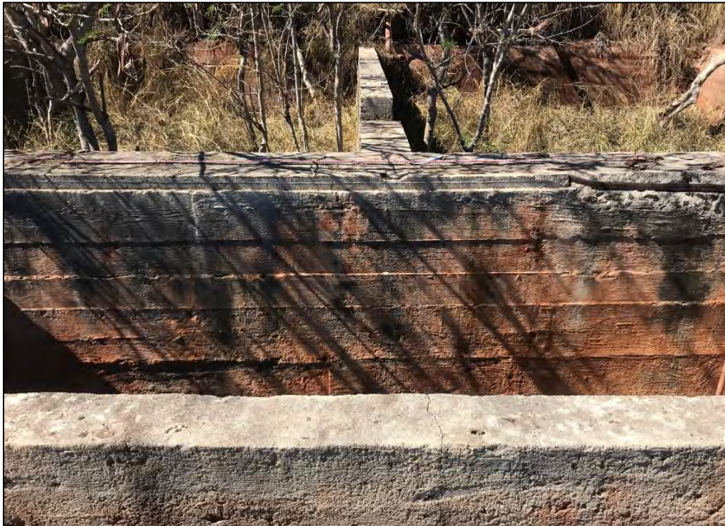
Figure 64. Overview of SIHP # 50-80-08-5593 Feature 2B, showing two large water storage compartments (background) and smaller compartment containing pipes and valves (foreground), view to northwest
