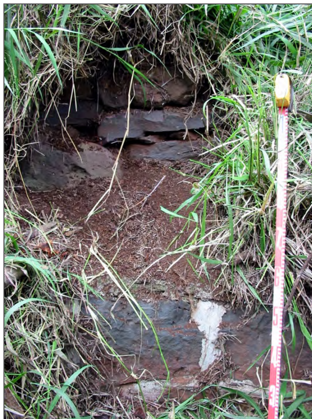
Figure 82. SIHP # 50-80-09-2268 showing the dressed basalt boulder and mortar Waiahole Ditch (top), and stacked basalt boulder and cobble retaining wall (below) (Tulchin and Hammatt 2004:53)
