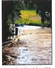
elevation to a level similar to the predicted level for a 500year flood discharge at the bridge. While the exact cause of the flow obstruction is not known, the likely culprit is again Hau Bush and associated debris. Clogged stream channels
