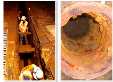
Nearly a quarter of the Kauai utility's water lines were installed more than half a century ago and there are still miles of pipe that date back as early as the 1920s.
