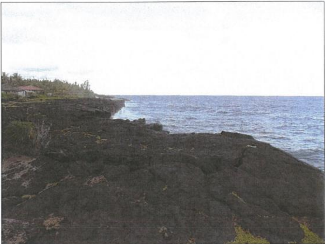
Figure 8. Bedrock shelf fronting the subject parcel at the coast, view to the north.
