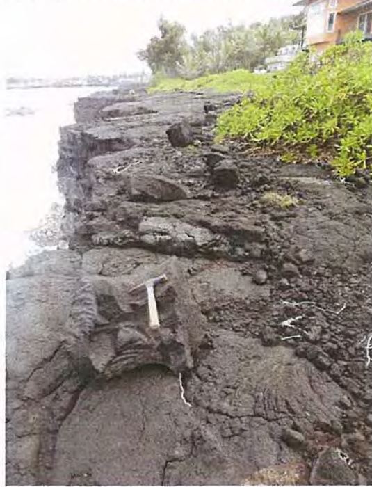
Figure 5. Photos of Sea Cliff in Front of Property
