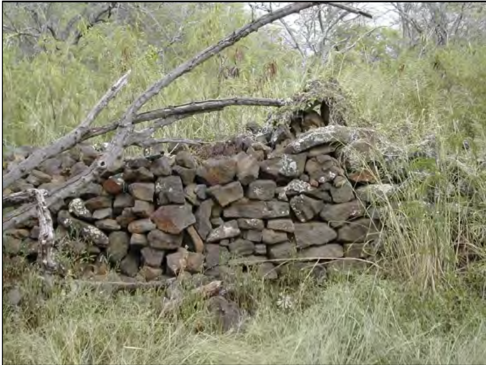
Figure 2-15. Portion of Kuakini Wall in project area.
