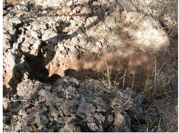
Figure 68. EU-24 base of excavation, view to the northeast.
