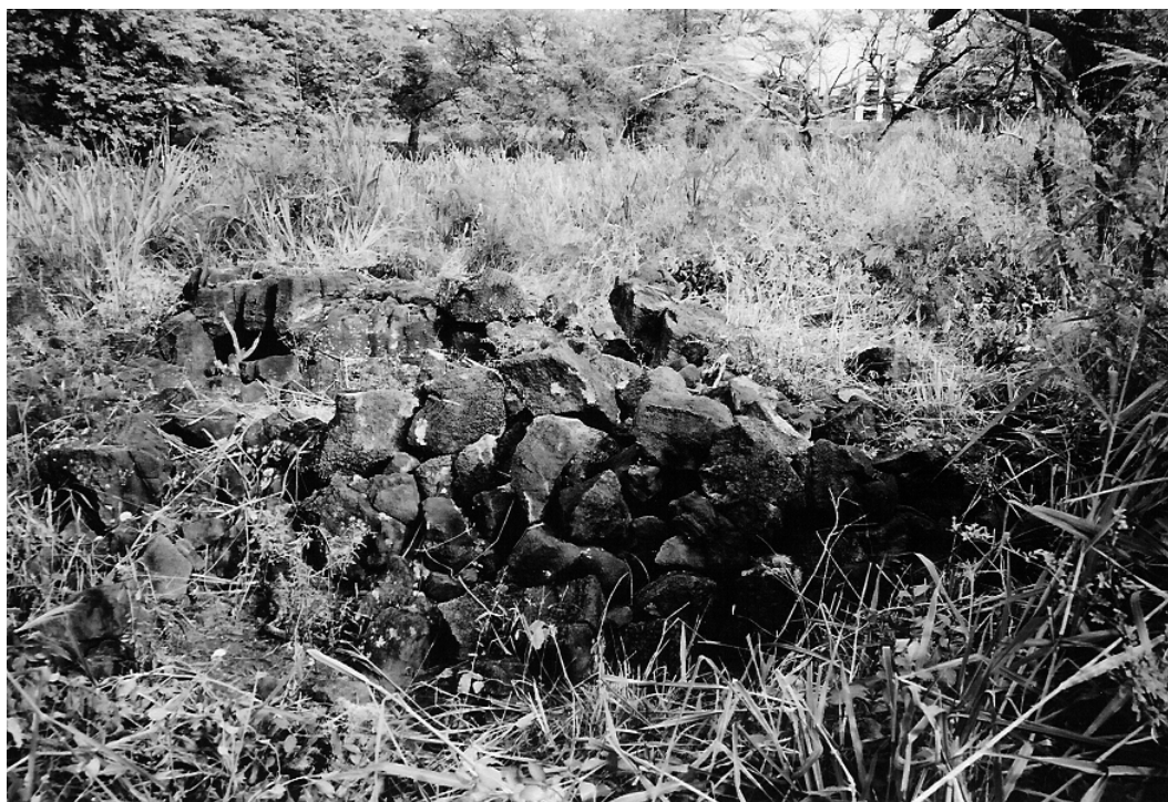
Figure 67. SIHP Site 23686 Feature 183 view to northwest.
