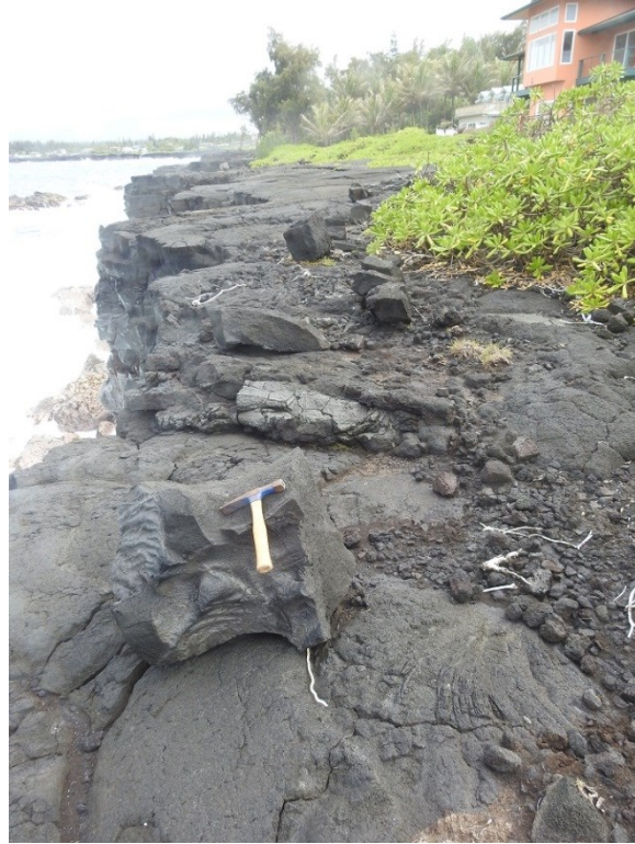
Figure 5. Photos of Sea Cliff in Front of Property
