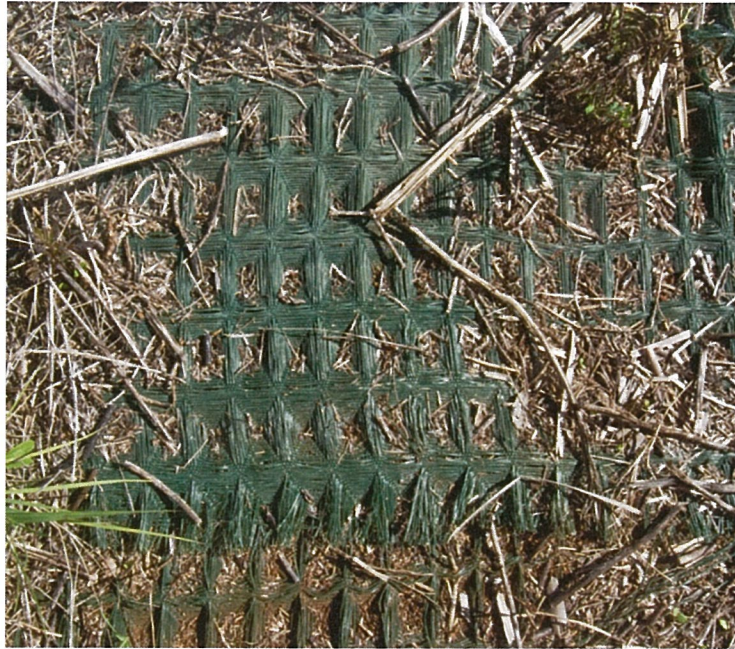
Figure 6. The geotextile “fabric” that covers several acres at and downslope of the former sugar-cane era reservoir.
