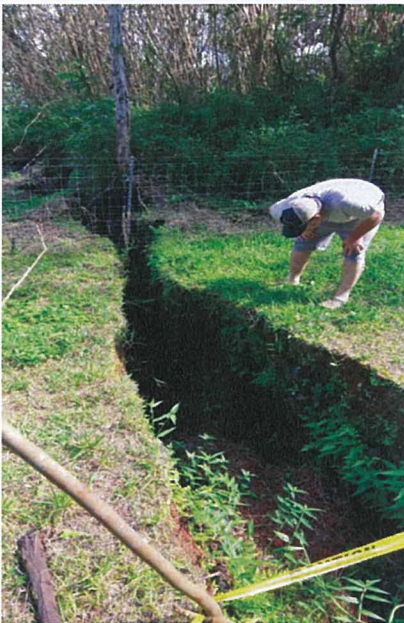
Photos 12 and 13. Crevices parallel to project access road.
