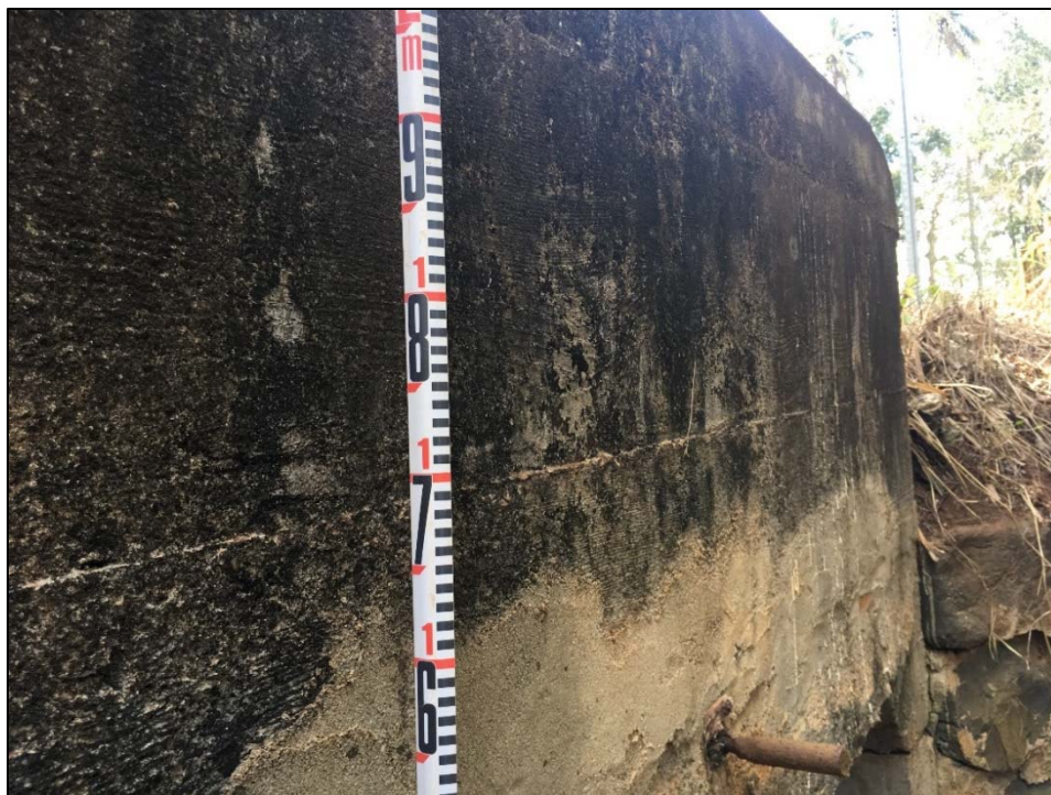
Figure 58. Photo of the west headwall of SIHP # 50-30-08-7021 Feature 5 showing wood grain pattern along headwall face and metal rod embedded in the concrete, view to southeast
