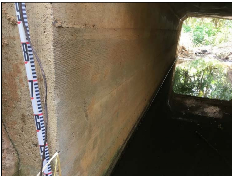
Figure 59. Photo of the north interior wall of culvert box of SIHP # 50-30-08-7021 Feature 5 showing wood grain pattern along the interior wall face, view to northeast
