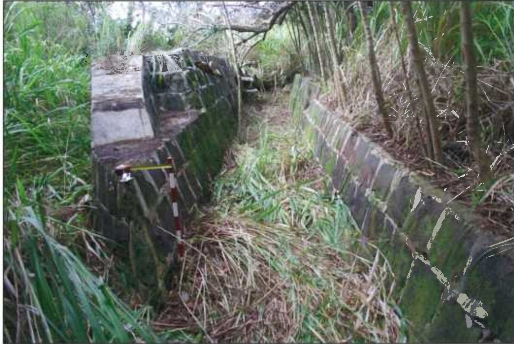
Figure 7. Cut basalt and mortar ditch (Feature 23, Site 2273) running parallel to Feature 22 and connecting with it by way of the sluice gate at Sub-feature A and the large opening to the left (tall grass) into Sub-feature B, view south; vertical scale bar is 80
