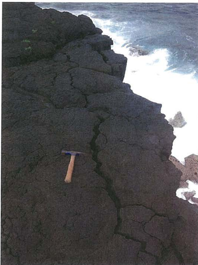
Figure 9. Extension cracks present at the Property's coastal cliff edge. These cracks, which are common along this stretch of coastline, develop as stresses are relieved at the cliff face, and contribute to the susceptibility of this upper pahoehoe flow to rare storm waves that impact the cliff face and force sea water into the horizontal contacts between flow lobes.
