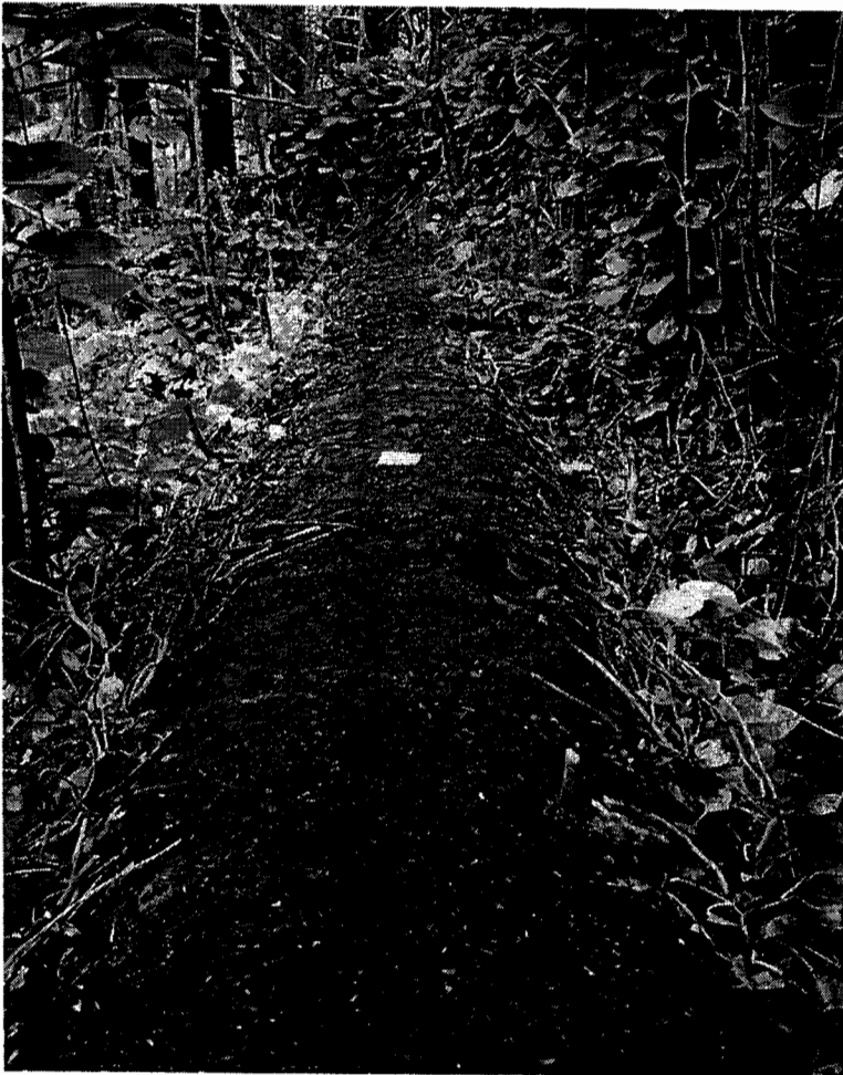
Figure 14. SIHP Site 24212 Feature 2, trestle abutment, view to the east.
