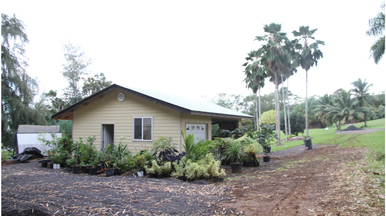
Storage and processing structure accessory to the agricultural uses of the Property on the Middle lot and early potted plant nursery area 2017
