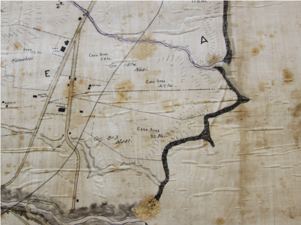
Exhibit 107, 1905 Historic pictures of the Property
