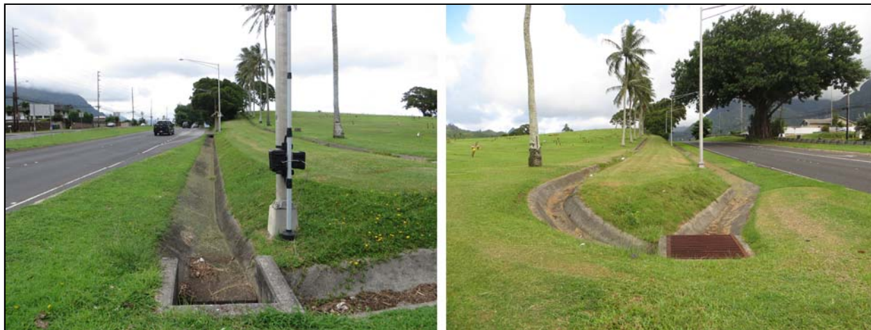
Northwest View of Drainage Facility Along Highway at HMP’s Main Entrance
