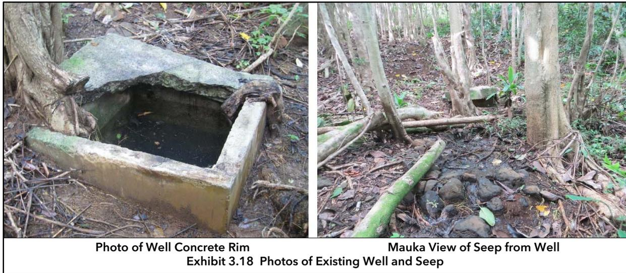
A small but perennial seep emerges about four feet downslope from the well (see Exhibit 3.18). Further down the waterway, the flowrate in the waterway continuously increases along the route to its ultimate discharge into the drain inlet at the end of Ohaha Place. Given the additions to the flowrate enroute downslope, it is more accurate to describe the seep as an area of discharge rather than a discharge from a single point (TNWRE, 2018).
