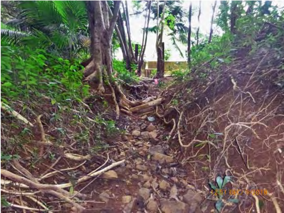
Figure 6. View towards the storm drain inlet from the incised channel.
