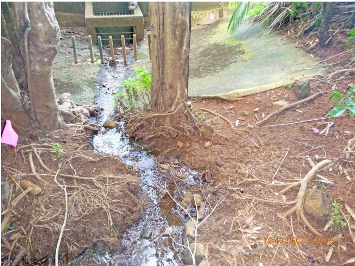
Figure 5. Flow from the perennial seep channel within the larger incised channel is directed to an inlet of the City and County storm drain system in Pikoiloa.
