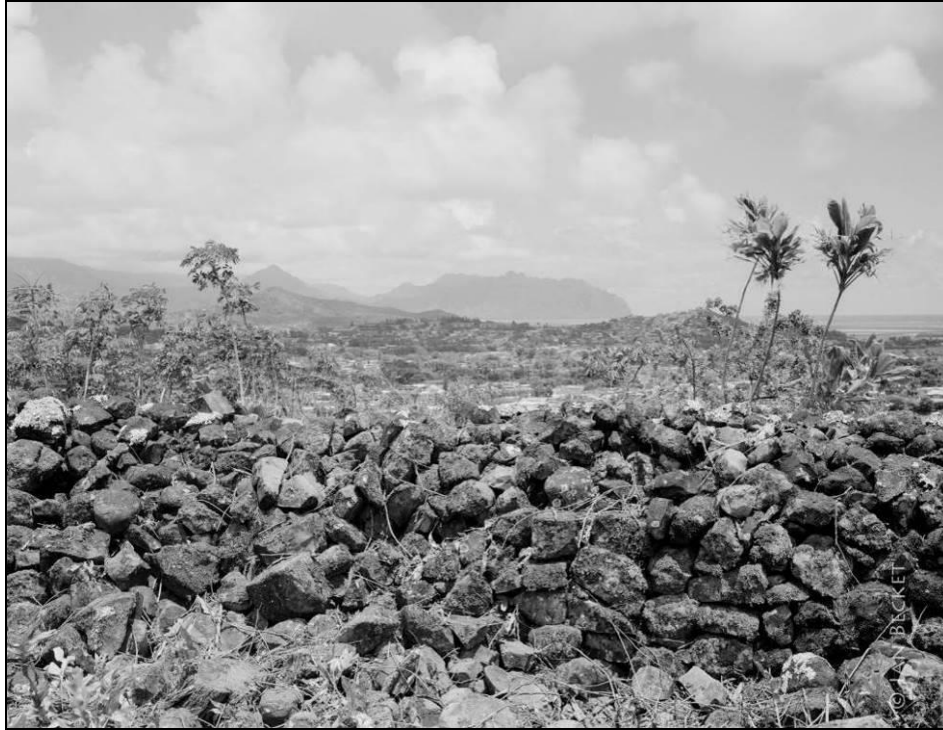
Figure 31. Photo of Kawa'ewa'e Heiau, view to north (Jan Becket 1995, permission of author)
