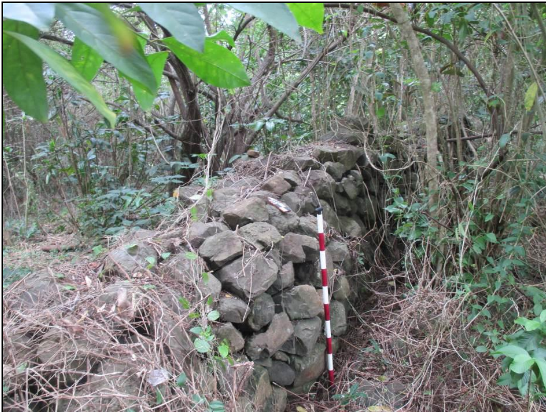
Figure 33. Photo within Kawa'ewa'e Heiau (SIHP # -354) showing the north interior wall (Feature 7) of the heiau in good condition, view northeast
