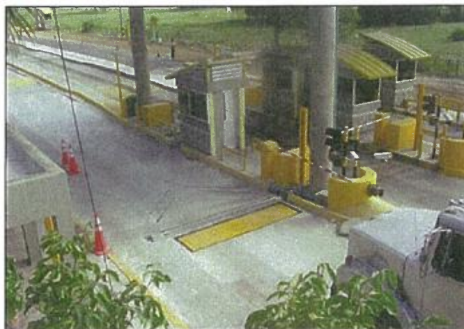
Figure 6.14 – Example of a Medium Speed, In-motion Axle Weighing System (Source: www.WorldHighways.com , 2014)
